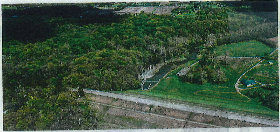
The Germantown Dam is one of five dams protecting residents and businesses in the five counties covered by the Miami Conservancy District. JIM NOELKER / STAFF
