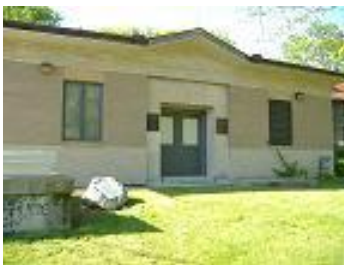
Springhouse Water Treatment Plant
