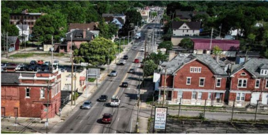
A section of North Main Street north of Great Miami Boulevard will be modified from four lanes to two, with a turn lane in the middle. STAFF
