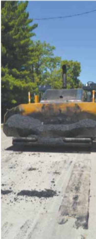
A work crew on Far Hills Avenue.
