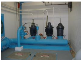
High Service Pumps at Springhouse
