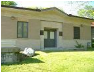
Springhouse Water Treatment Plant
