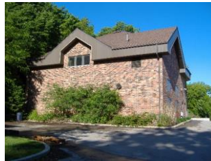
Shafor Water Treatment Plant
