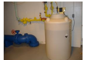
Chlorine Pump at Springhouse
