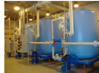
Softening Units at Shafor Water Treatment Plant
