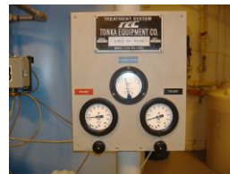
Control Panel at Springhouse
