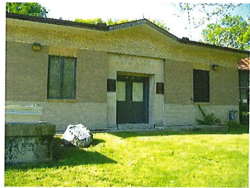
120 Springhouse Water Plant
