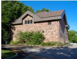
Shafor Water Treatment Plant
