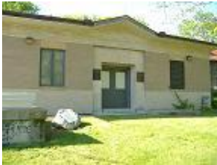
Springhouse Water Treatment Plant
