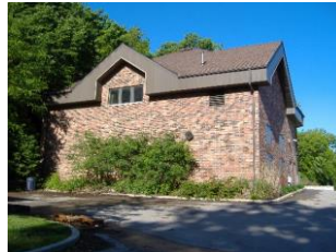
Shafor Water Treatment Plant
