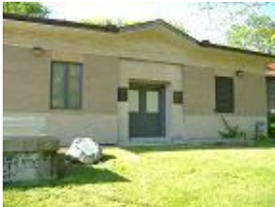
Springhouse Water Treatment Plant
