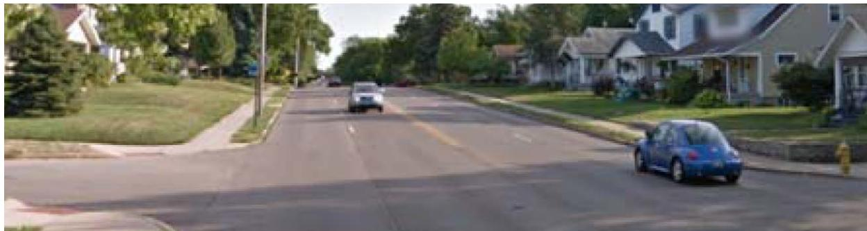
The typical section of Shroyer Road averages 44 feet between the face of existing curbs. Sidewalk (5 feet wide) exists on both sides of Shroyer Road. The tree lawn varies between 2 and 3 feet wide within the majority of the study area. The pavement wearing surface is asphalt but the roadway base is concrete. Joint failures of the concrete result in cracking of the asphalt surface which requires sealant.
