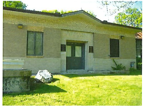
120 Springhouse Water Plant
