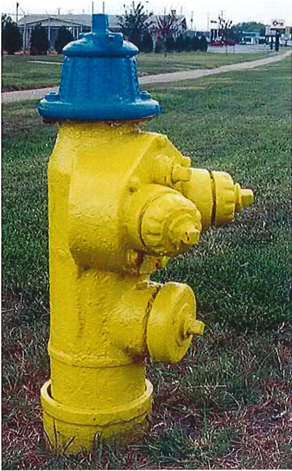
OLDER "BOURBON" TYPE HYDRANT
