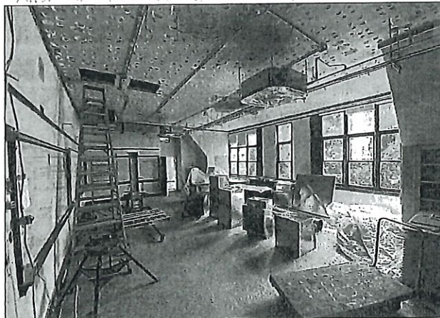
Classrooms in Oakwood High School/junior high are receiving new heating and air conditioning systems as part of an $18 million renovation project. CONTRIBUTED PHOTOS
