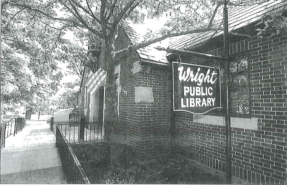
Wright Memorial Public Library is on the National Register of Historic Places. STAFF
