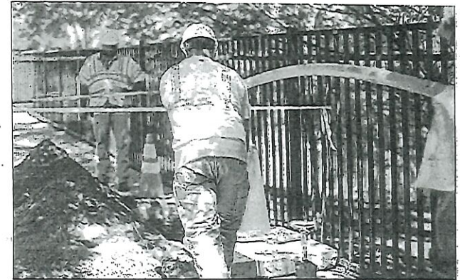
Crews worked to install the Miami Valley Communications Council's fiber optics network last year in Centerville. Trotwood officials are seeking federal funds to help tap into the network. FILE
