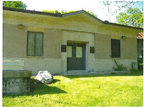
120 Springhouse Water Plant
