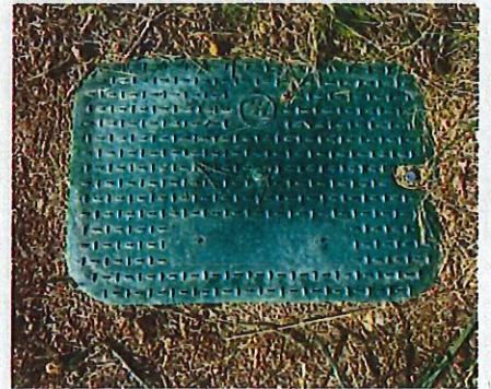
Handhole Fiber Junction Box Size: Flush-mounted and Inground Number of boxes in Oakwood: Approximately 2,000
