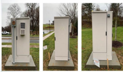
Distribution Hub Cabinet
