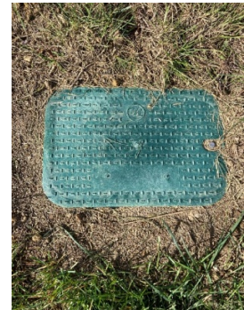
Handhole Fiber Junction Box
