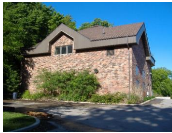
Shafor Water Treatment Plant
