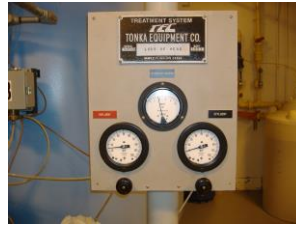
Control Panel at Springhouse
