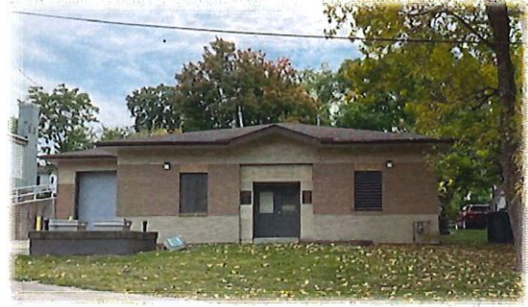
120 Springhouse Water Plant
