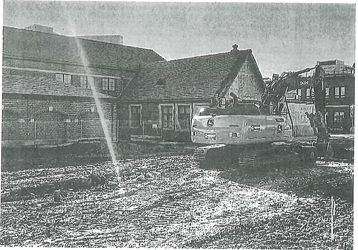
Progress continues on the future site of the Rick and Jane Schwartz Performing Arts Wing at Oakwood Junior and Senior High. Work started Dec. 21.
