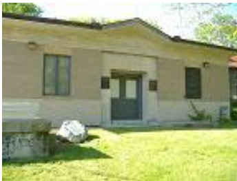
Springhouse Water Treatment Plant
