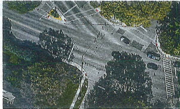
A roundabout is being examined for the six-spoke intersection involving Oakwood Ave., Thruston Blvd. and Far Hills Ave. The intersection is just south of Dayton on Ohio 48 as you climb the hill to Oakwood. JIM NOELKER/STAFF
