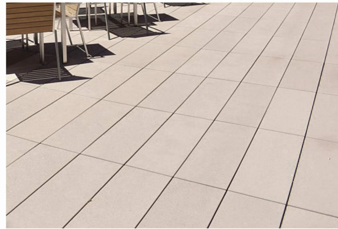
P7 CONCRETE PAVER - TYPE 5 MATERIAL: PRECAST CONCRETE, PEDESTAL SET SIZE: 18" X 48" COLOR/FINISH: LIGHT BUFF/TAN, SANDBLAST
