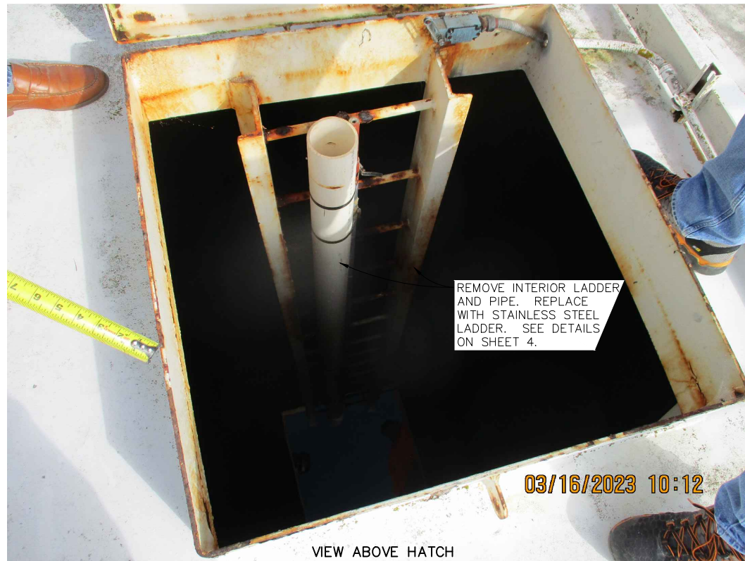
VIEW ABOVE HATCH
