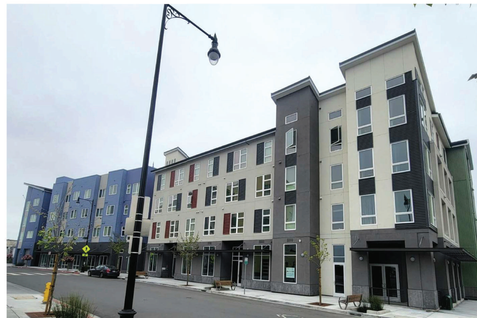
View from south of Project Site looking west at 4-story La Via Apartments at 350 N. Water Street.
