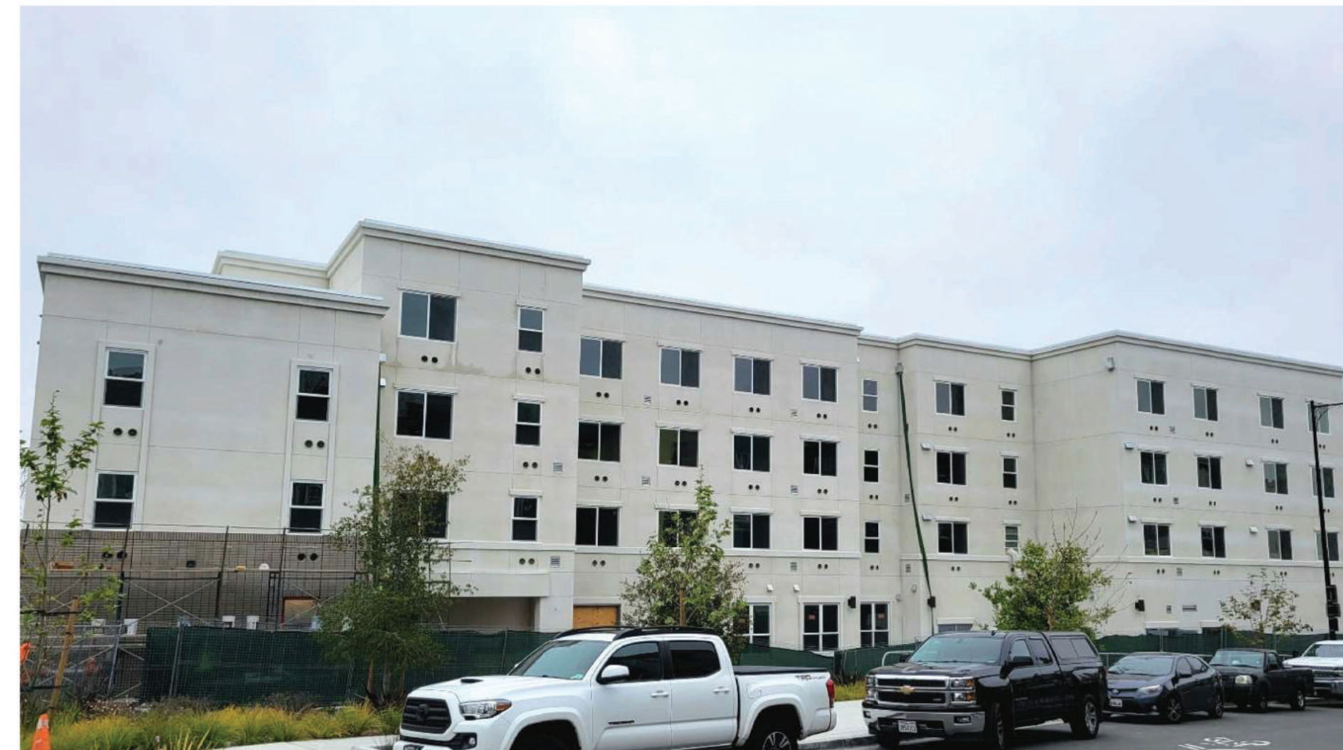
View from south of Project Site looking north at 4-story PBN 414 Apartments at 414 Petaluma Blvd. North.
