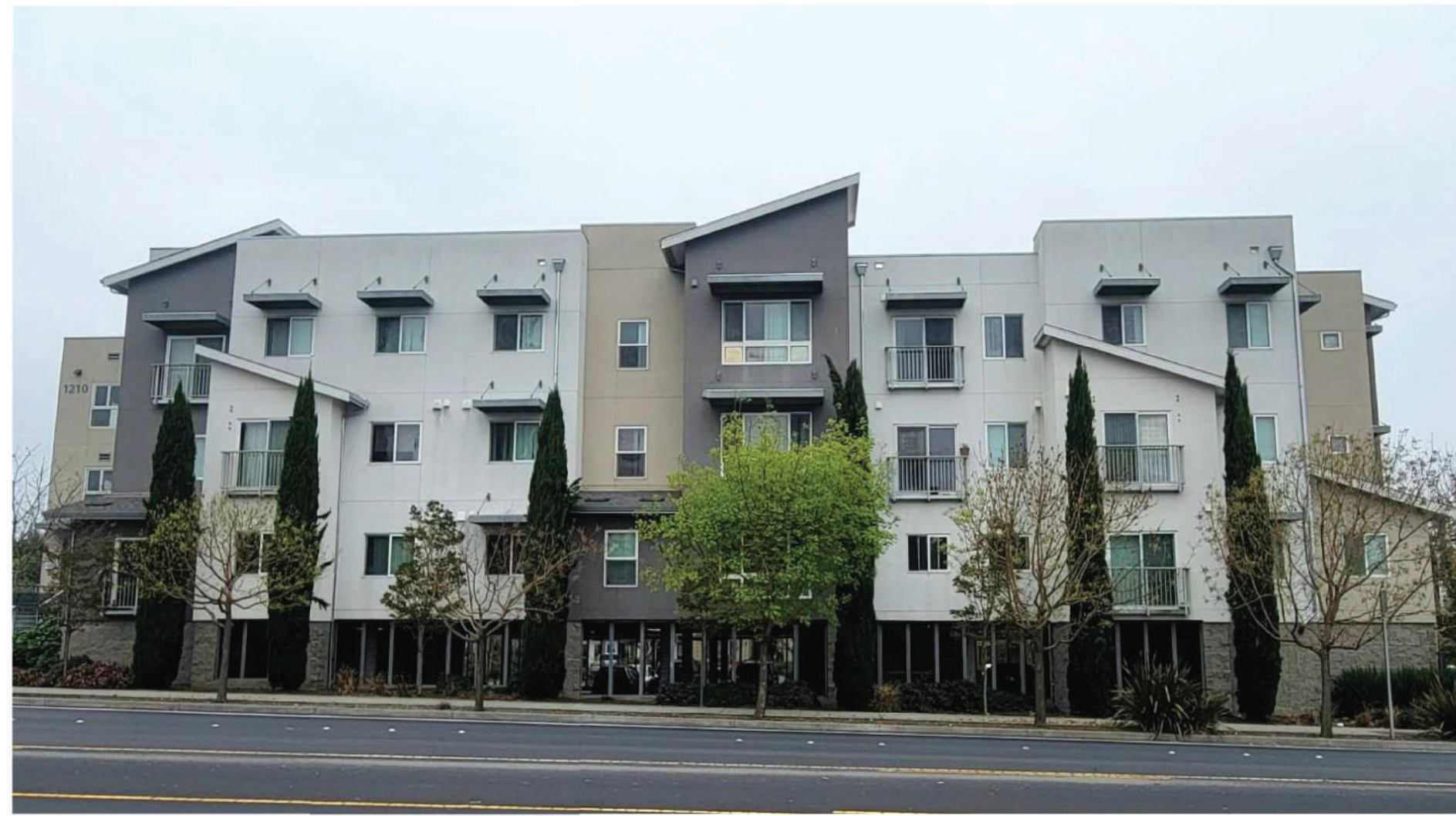
View from Project Site looking east at 4-story Logan Place Apartments at 1210 Petaluma Blvd. North.
