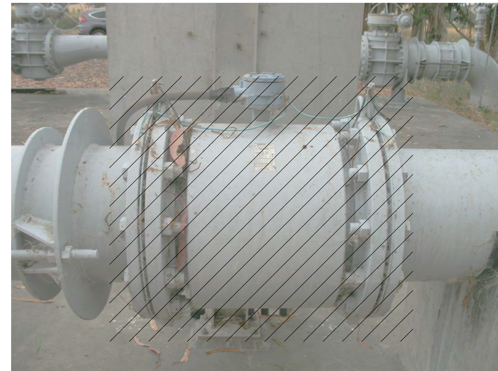
(E) (E) FLOWMETER FIT-1105 REPLACEMENT (2)(4) SCALE: NTS
