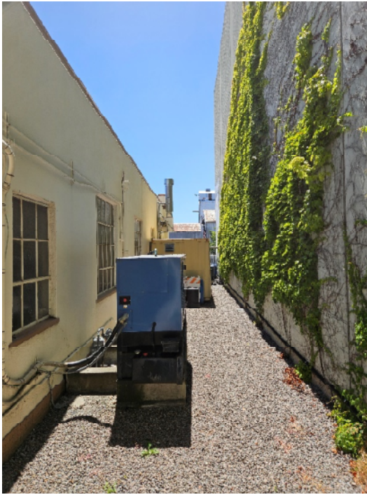
Limited view of North Side Yard – Source: Report Author
