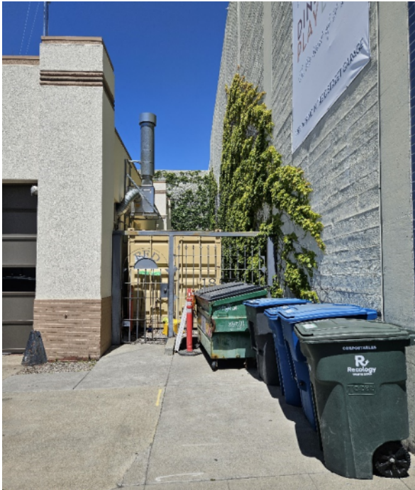
Current trash storage facing D street public way – Source: Report Author
