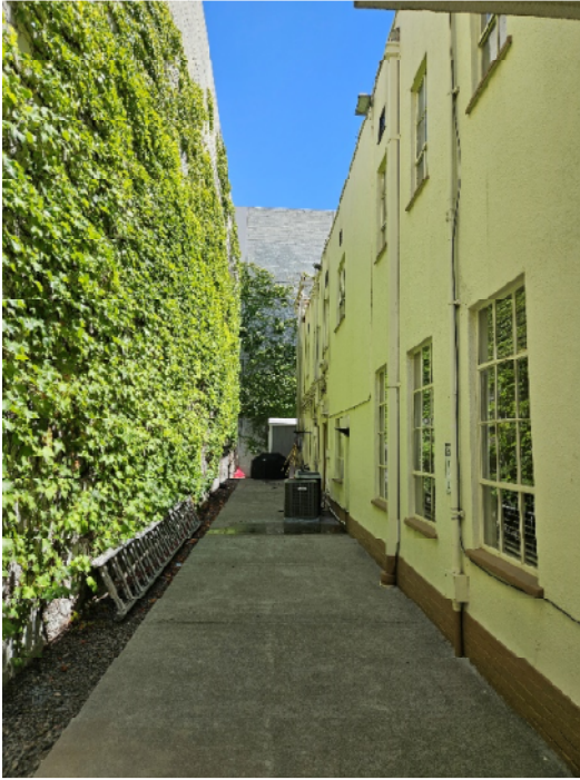
Interior view of West Side Yard – Source: Report Author
