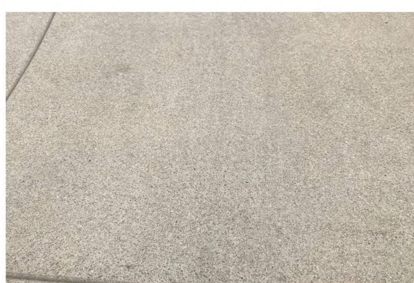
P1 C.I.P. CONCRETE PAVEMENT MATERIAL: CAST-IN-PLACE CONCRETE COLOR: STANDARD GREY FINISH: TOPCAST #05 "SANDBLAST" JOINT: SAWCUT
