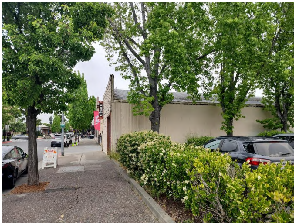
Photograph 9. Ancillary building, east elevation, view west (FCS 2024)
