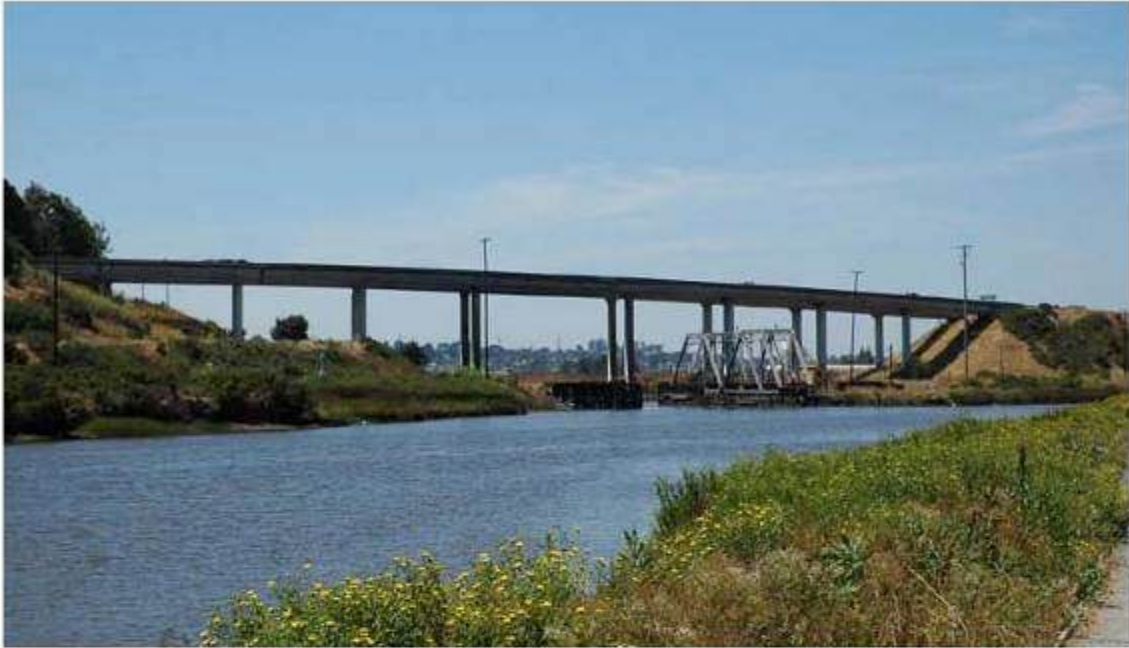
Figure 3.1-39 Existing Petaluma Bridge Looking East
