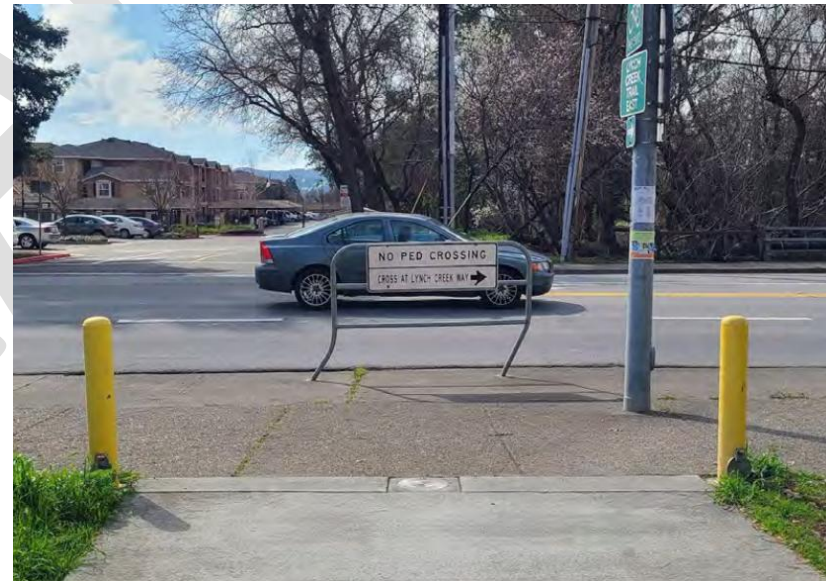
Absence of a trail crossing on Lynch Creek Trail at North McDowell Boulevard. This is also a location where the City removed the middle bollard to improve trail accessibility.
