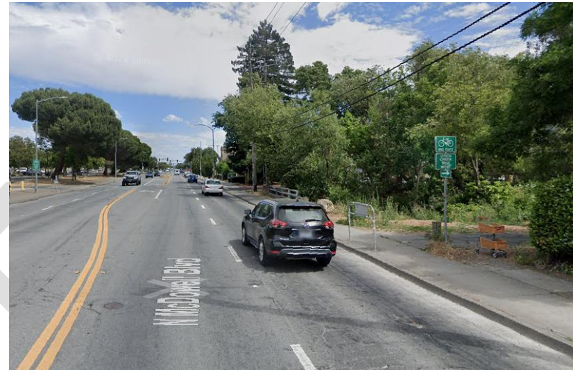
The Lynch Creek Trail, Petaluma's primary east-west trail, lacks convenient access and crossings where it intersects N. McDowell Boulevard and Sonoma Mountain Parkway
