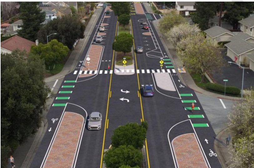
Lane conversion projects enable underutilized vehicle lanes to be reallocated for other uses, including walking, bicycling, parking, and greenery
