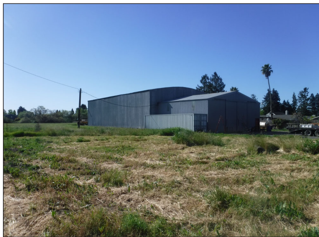
PHOTO 3: Existing warehouse/workshop building on site.
