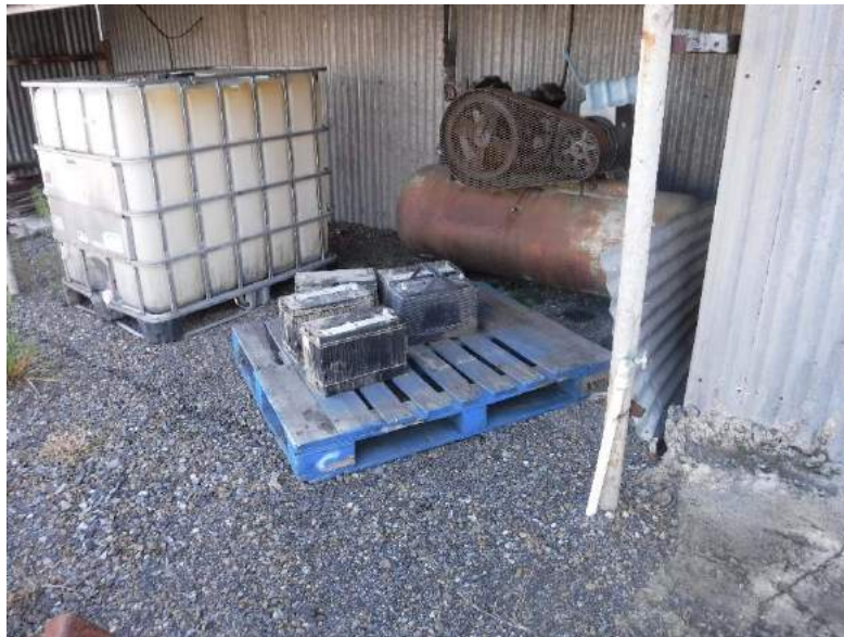
Photo 12: Liquid storage, an air compressor, and electrical batteries located under the storage roof attached to the southwest exterior side of the shop.
