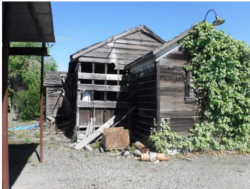
Photo 6: Back of abandoned residence near the southwest property line of the Subject Property.
