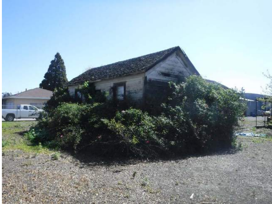
Photo 7: Front of abandoned residence shown in Photo 6.
