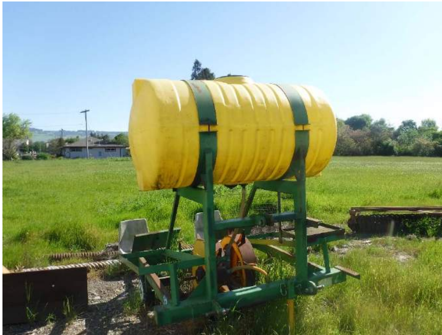
Photo 1: Above-ground storage tank mounted on trailer behind workshop. Empty, with some staining or residue on the bottom interior of the tank.
