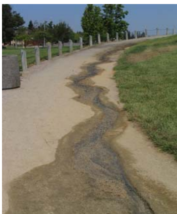
Water run-off has damaged the urban separator trail near airport.
