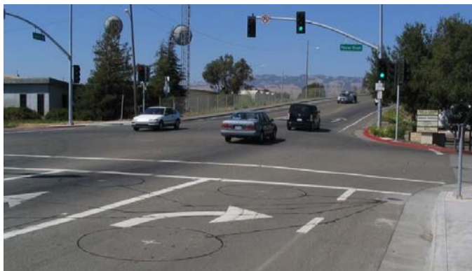
This scene at the intersection of Caulfield Lane with Payran Street is not uncommon. A bicycle push button is located on the far right side at the curb - an inconvenient location for bicyclists wanting to travel straight or turn left.
