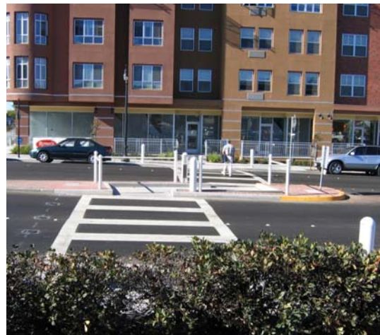
The pedestrian corral on Washington Street includes in-roadway warning lights.
