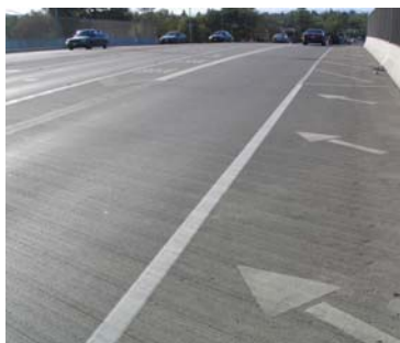
An interchange in Davis, CA, has pavement markings signaling bicyclists when to merge left to the other bike lane. This location also had signage.
