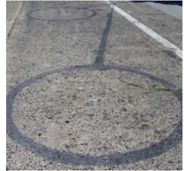
Round loop detector sawcut.
