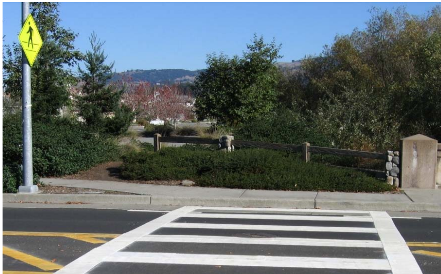
Corona Creek Trail at Ely Road: no curb ramp on one end of crosswalk, the trail entrance is on Fieldstone Lane, and landscaping and a berm make it difficult to see that there is a trail on the other side.
