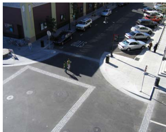
Bulb-outs such as these at the intersection of C and Second Streets are prevalent in the new Theatre District.
