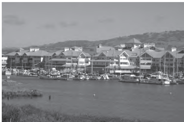
The 198-berth Petaluma Marina was constructed in 1987.
