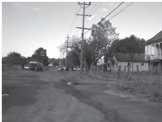
Unfinished street cross-sections, such as this segment of Shasta Avenue shown above, create opportunities to implement new street types at such time as these streets are fully improved with curb, gutter, landscape strips and sidewalks.
