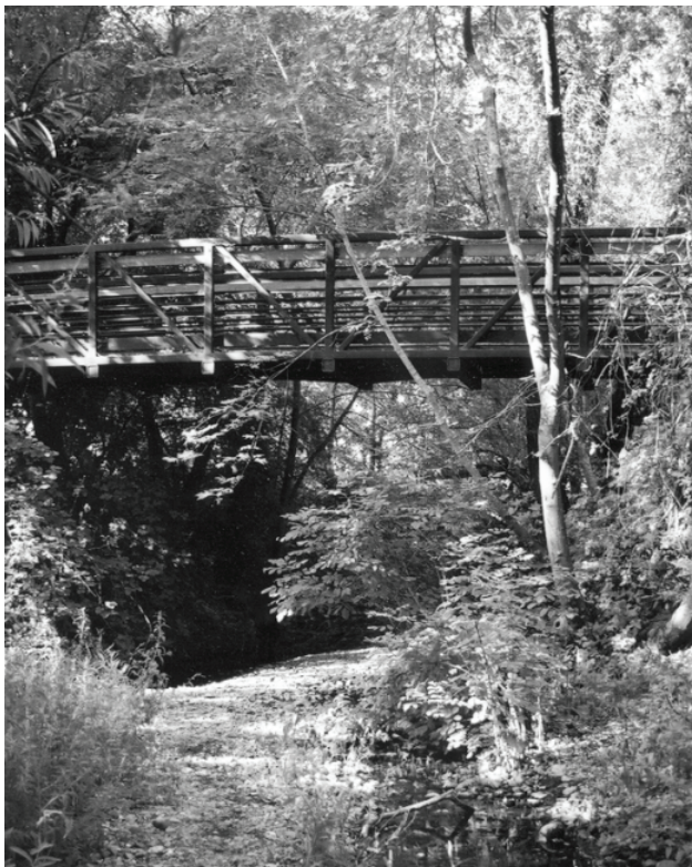
A multi-use trail bridges over Lynch Creek.
