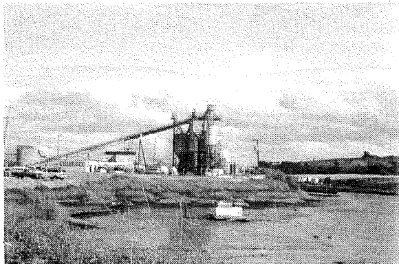
Retention of river dependent industries and their barge traffic is a priority in the Downstream Segment , as well as acquisition of McNear Peninsula (on the right) for a park and marsh restoration.
