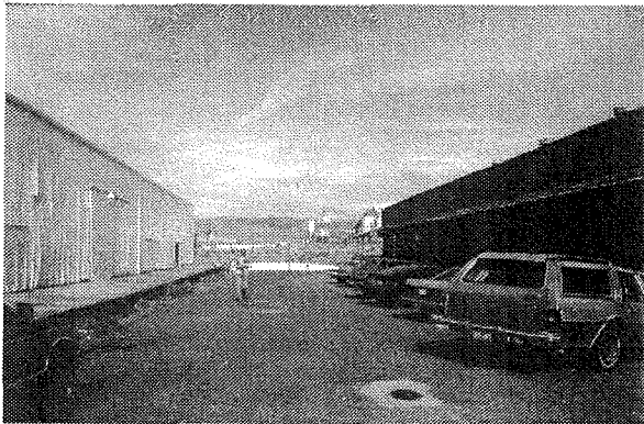
Access to the riverfront trail will be provided at public streets that terminate at the river wherever feasible, such as at the end of "G" Street, in addition to the staging areas.
