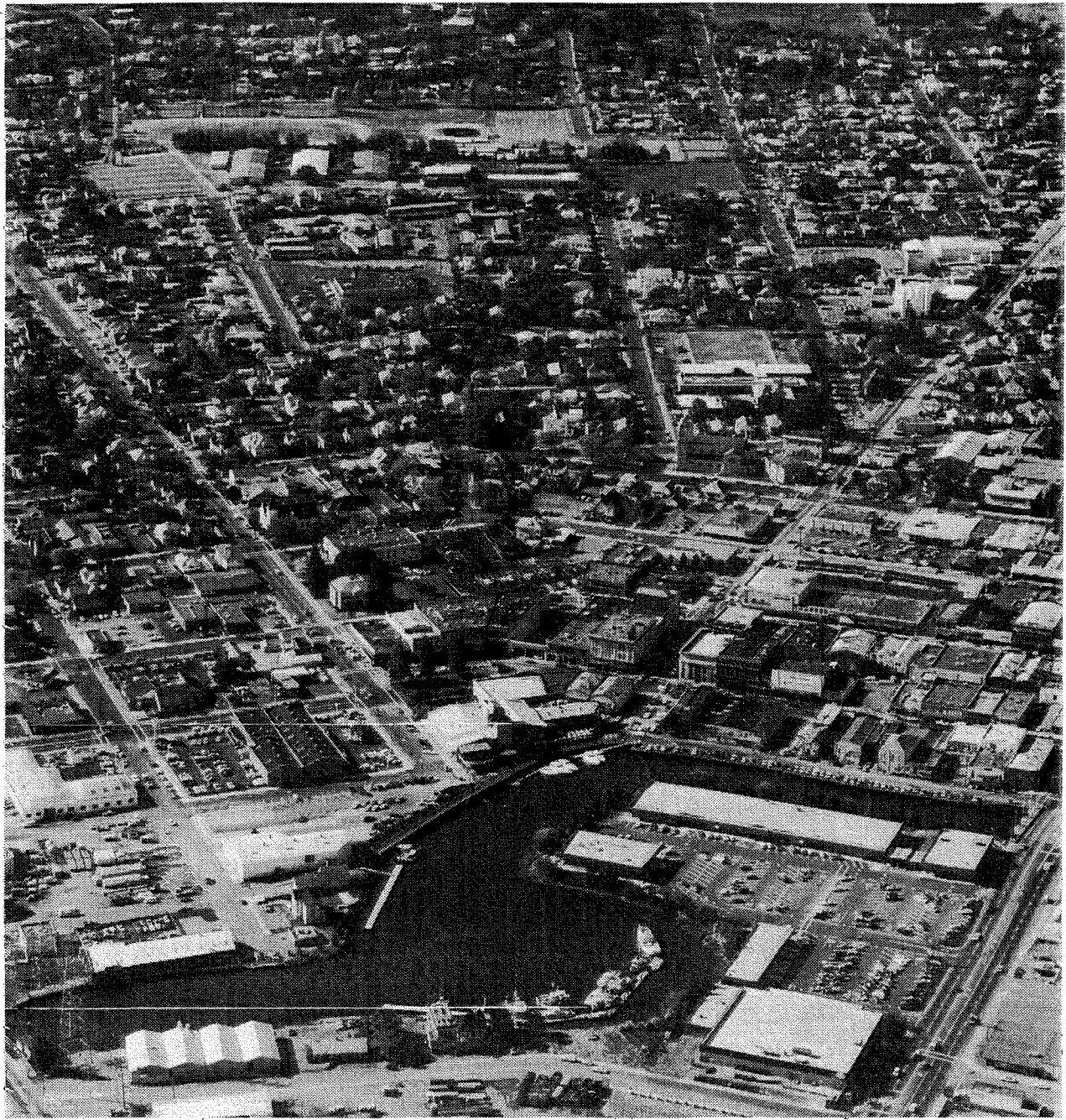
Downtown Petaluma at the Turning Basin of the Petaluma River looking southwest, 1986. Activating and revitalizing the downtown waterfront is the centerpiece of the River Plan.
