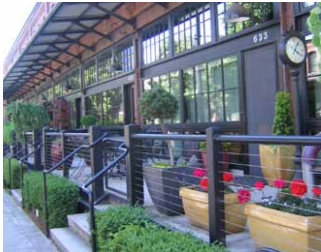
A raised Dooryard provides separation for a flexible area that contains a mix of ground floor residential and office.
