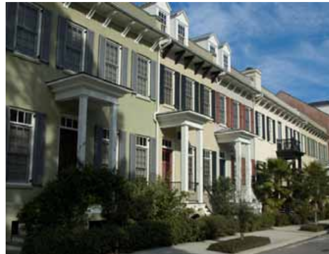
2 1/2 story townhomes with side loaded stoops and landscaped setback. The townhomes have a simple facade plane with detailing at the stoops, windows, and eaves.
