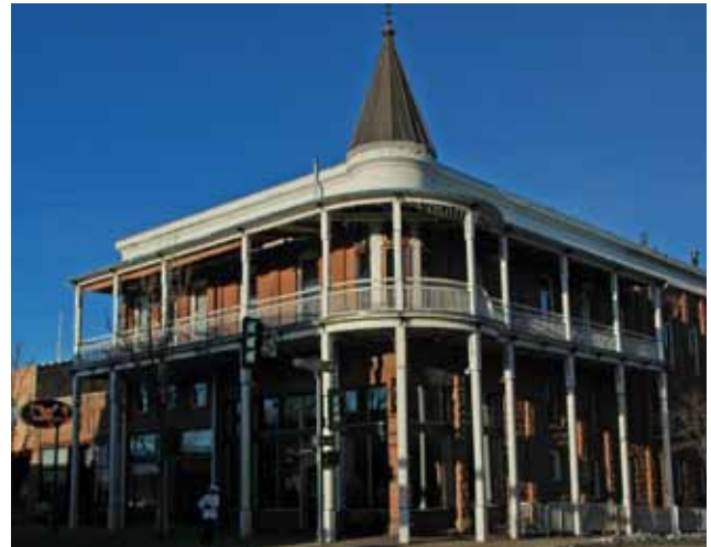
A wrap-around Gallery with a covered second level. The upper level should not be used as the only means of circulation.
