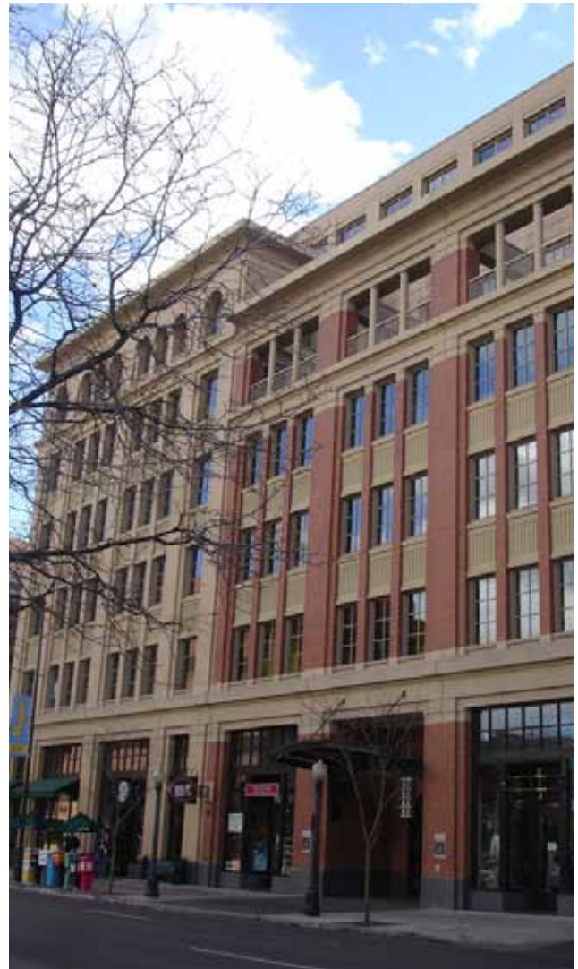
Another view of the Mid-Rise building above. The change of materials and eave line break up the scale of the building.
