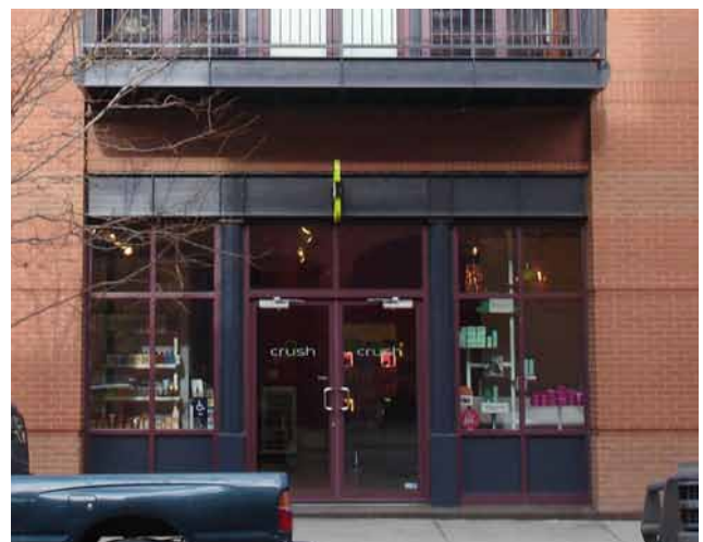
The Shopfront has a high percentage of glazing allowing for the passing pedestrian to view a store's merchandise.
