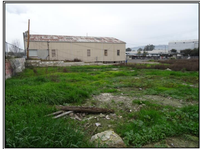
Looking north across the remnant concrete foundations and at Structure A.
