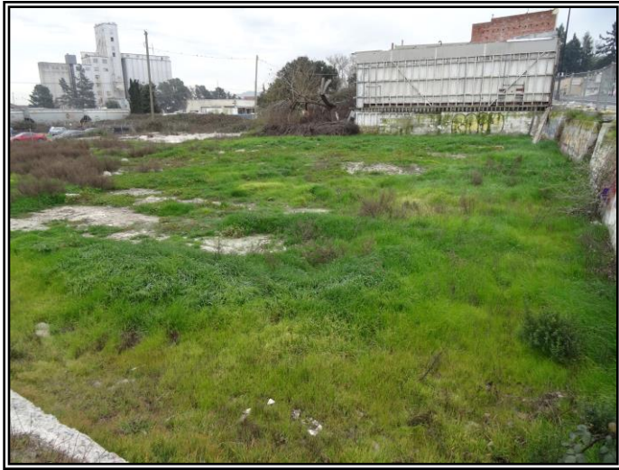
Looking south at the remnant concrete foundations of the former Structures J and S.
