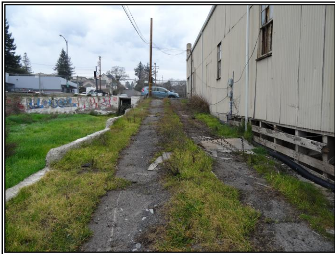
Looking west along the southern wall of Structure A.
