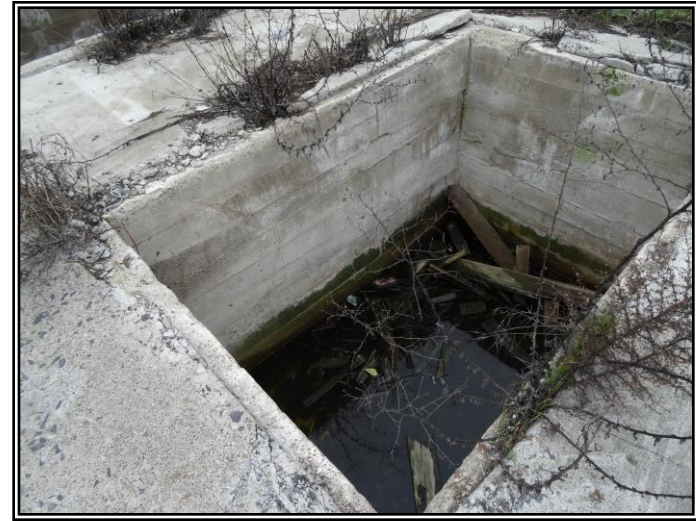
Looking at an opening in the remnant concrete foundation.
