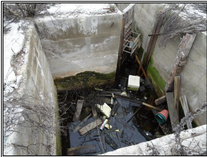
Looking at a second opening in the concrete foundation.
