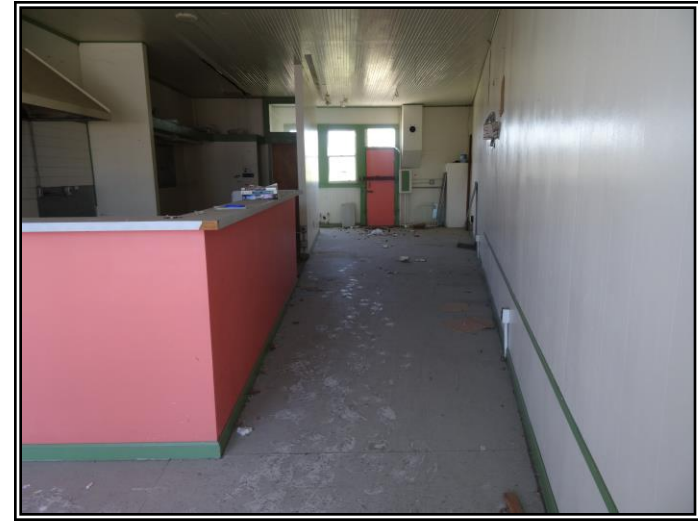
Looking at the interior of Structure CC/DD.
