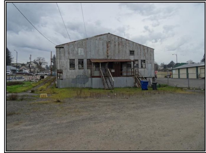
Looking west at Structure A located on the northwestern portion of the Site.
