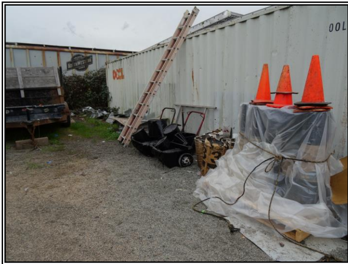
Looking at the storage of roofing materials and equipment.
