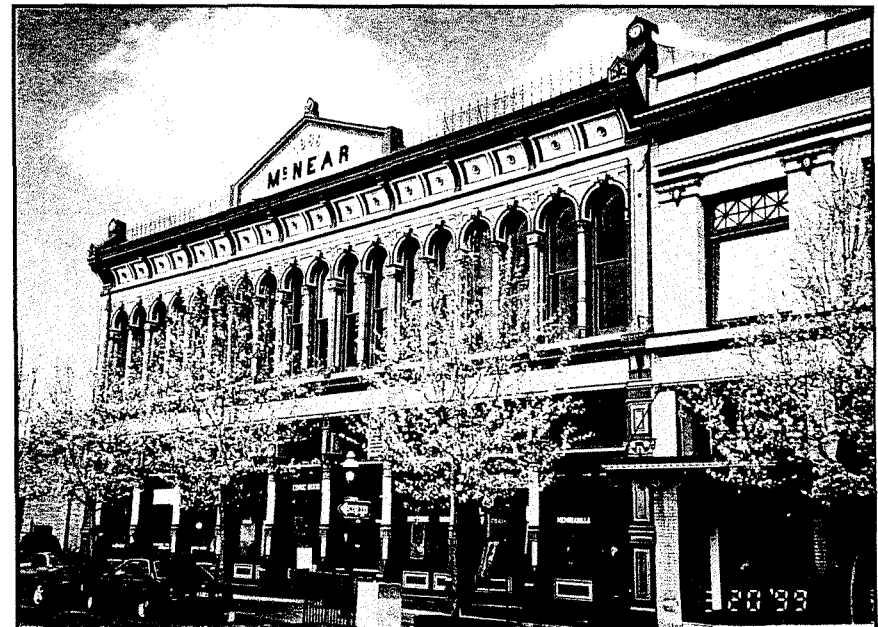
McNear Building, 1886 Kentucky Street
