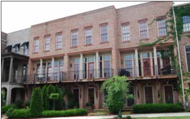
A series of townhouse units lining a small open space.
