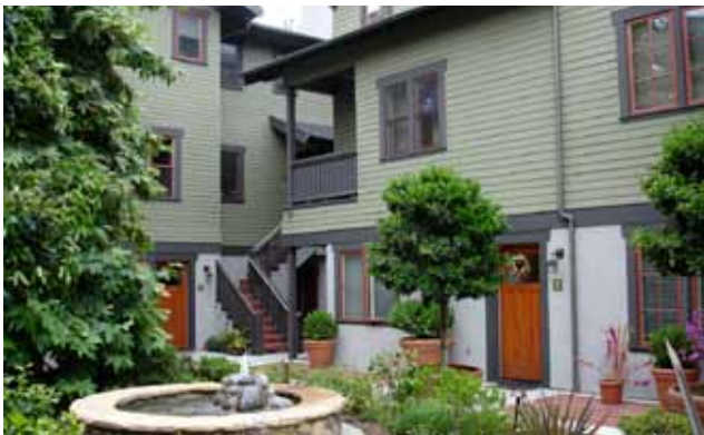
A courtyard defined by two and three story buildings.
