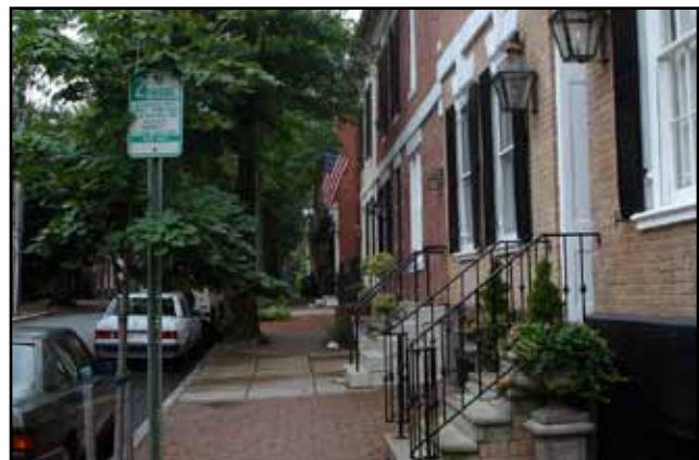
These stoops on townhouses with slightly recessed entries and a minimum setback allow the steps to engage the street.
