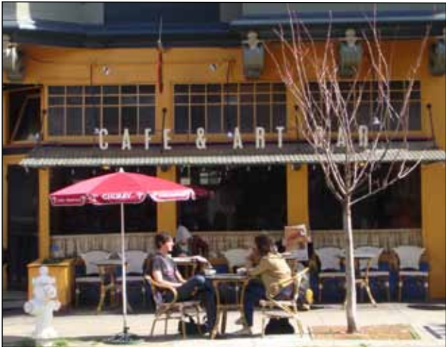
Projecting signage on a metal awning.
