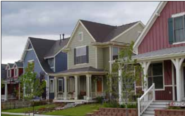
Newly constructed two-story cottage houses
