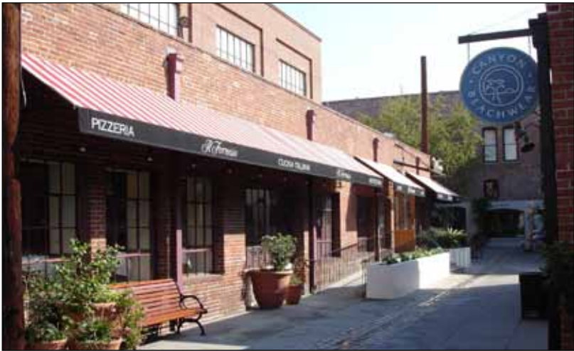
Series of awnings along a frontage.
