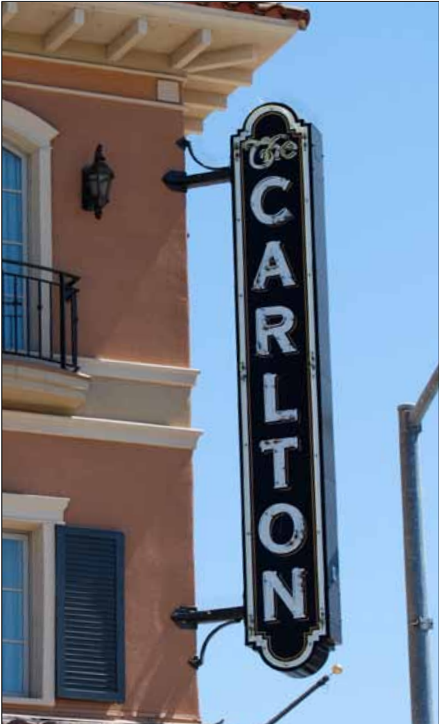
Marquee sign at corner terminating at eave.
