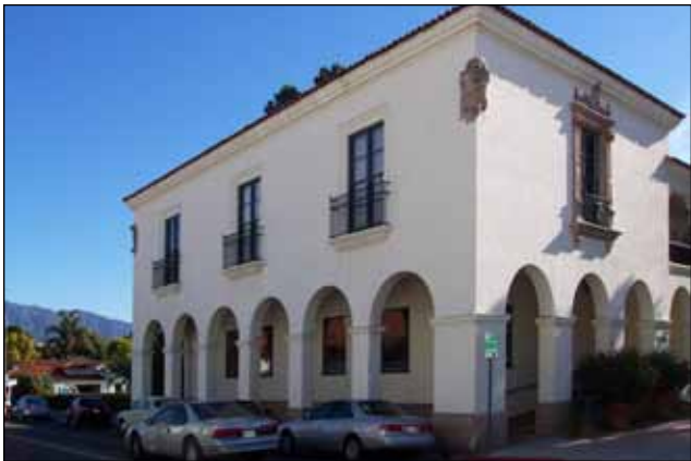
An example of an arcade encroaching the public ROW. The arcade provides the only means of circulation along the ROW.
