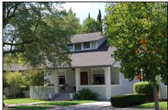
Projecting porch integrated into the overall massing
