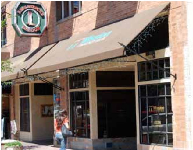
Awning with decorative supports and open end.
