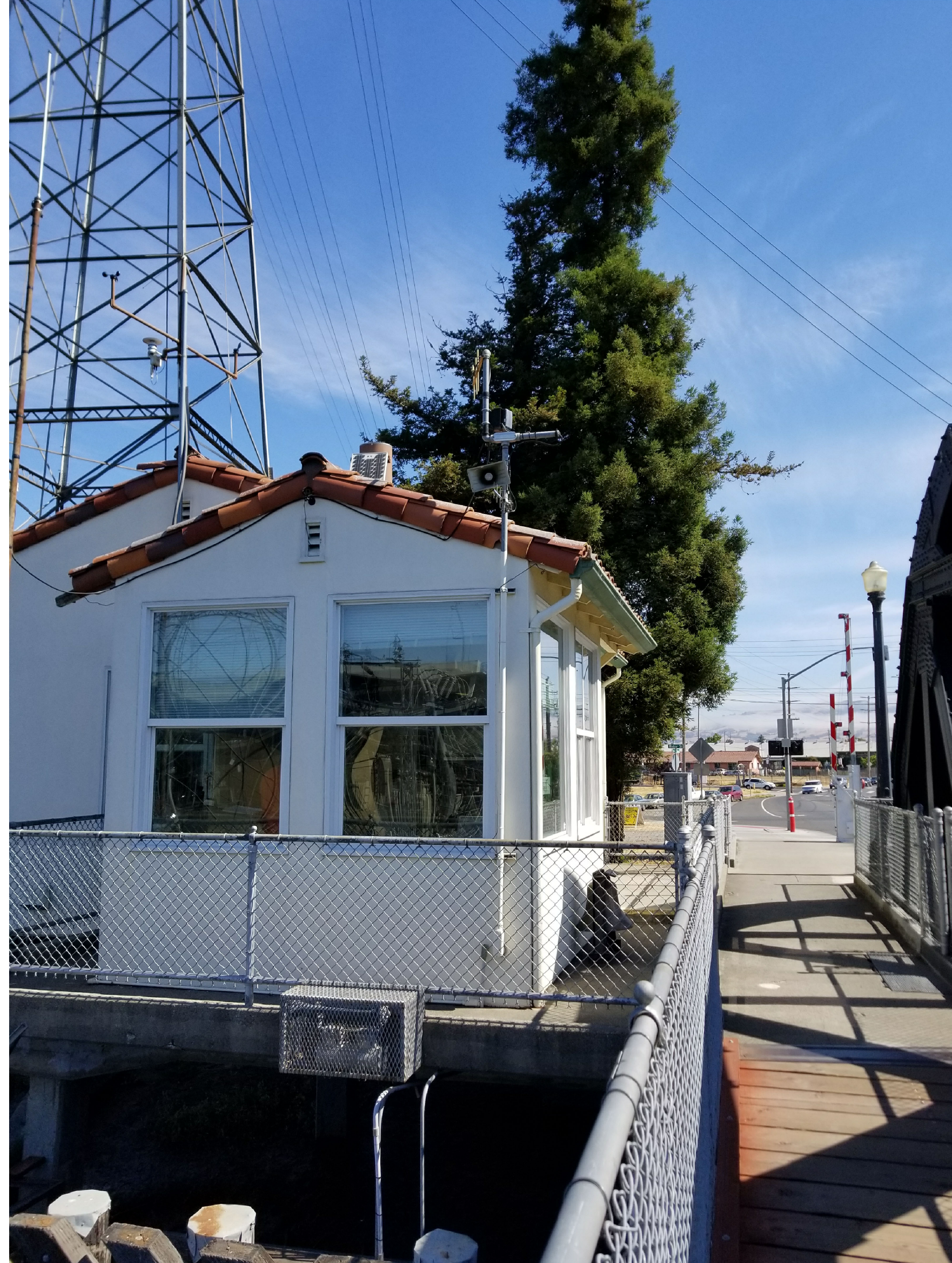
TENDER HOUSE SOUTH VIEW
