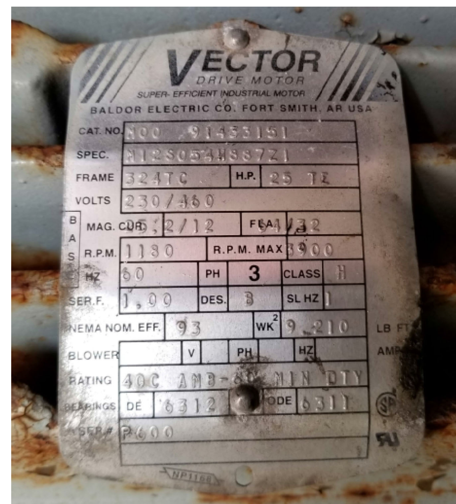
EXISTING MAIN SPAN MOTOR NAME PLATE
