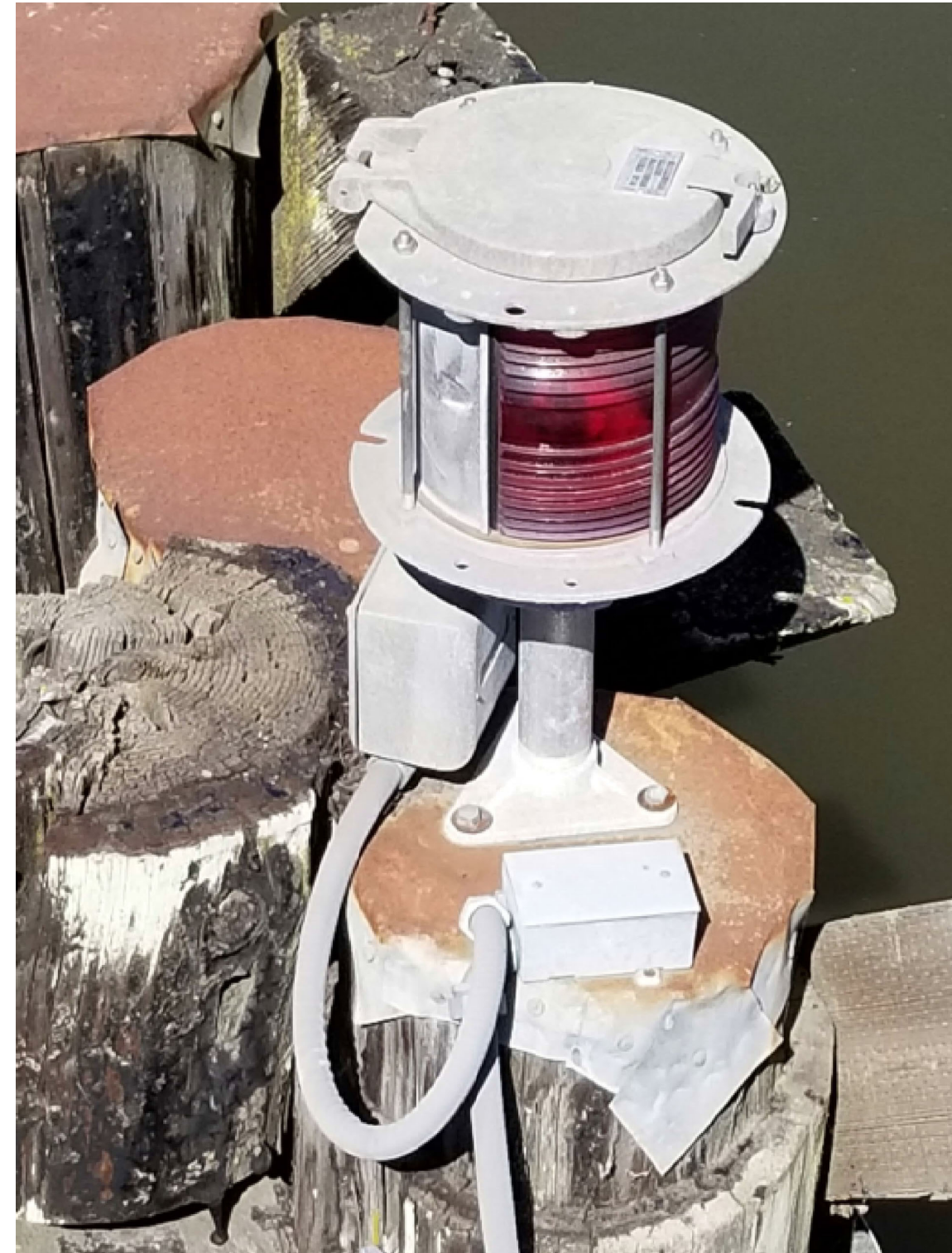
TYPICAL FLEX CONDUIT AT NAVIGATIONAL LIGHTS
