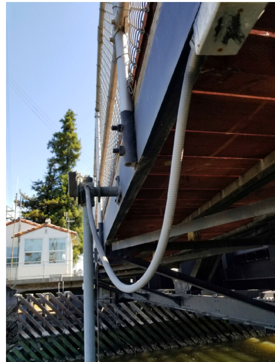
TYPICAL FLEX CONDUIT AT NAVIGATIONAL LIGHTS
