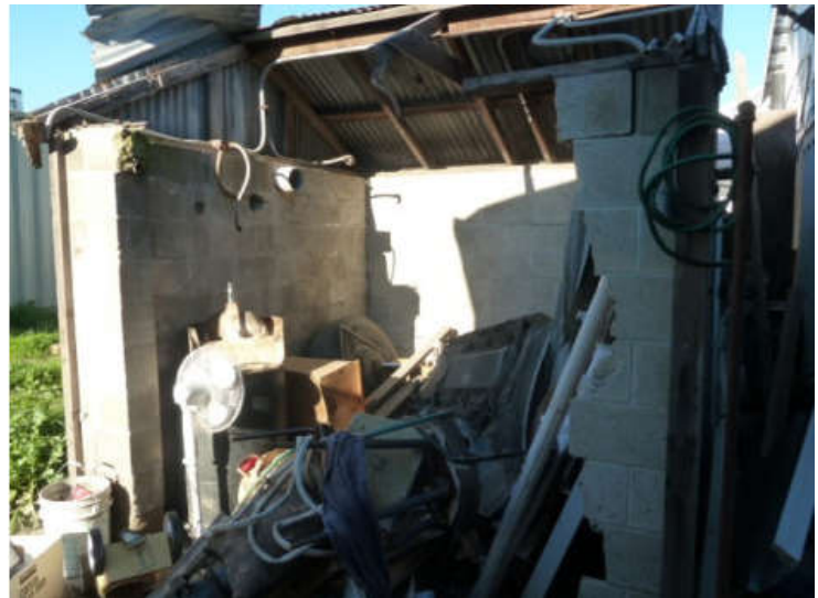
Photo #44: Interior former boiler shed
