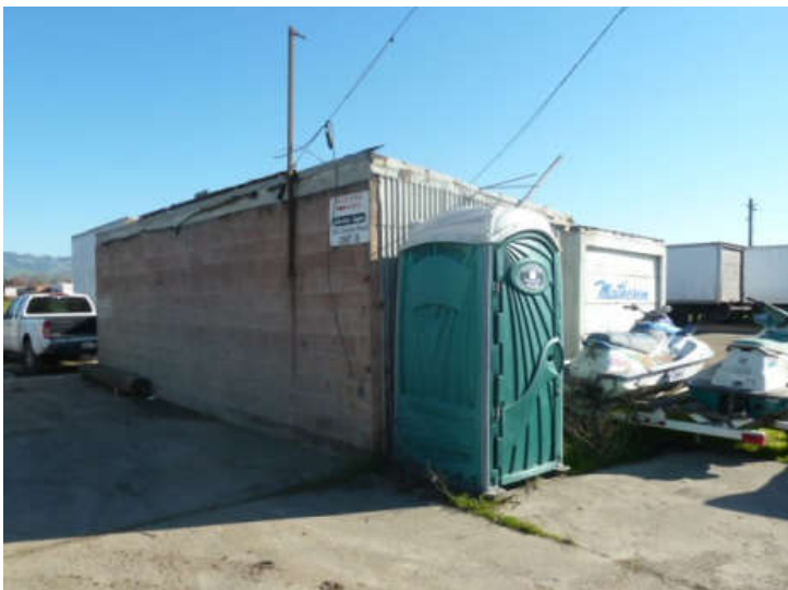
Photo #42: Masonry storage shed (locked)
