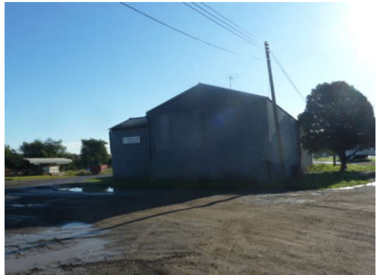
Photo #29: Central metal building associated with truss manufacturing business (view to east)
