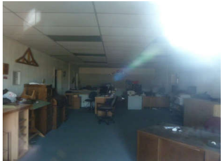
Photo #32: Office area of central metal building associated with truss manufacturing business (locked during visit)
