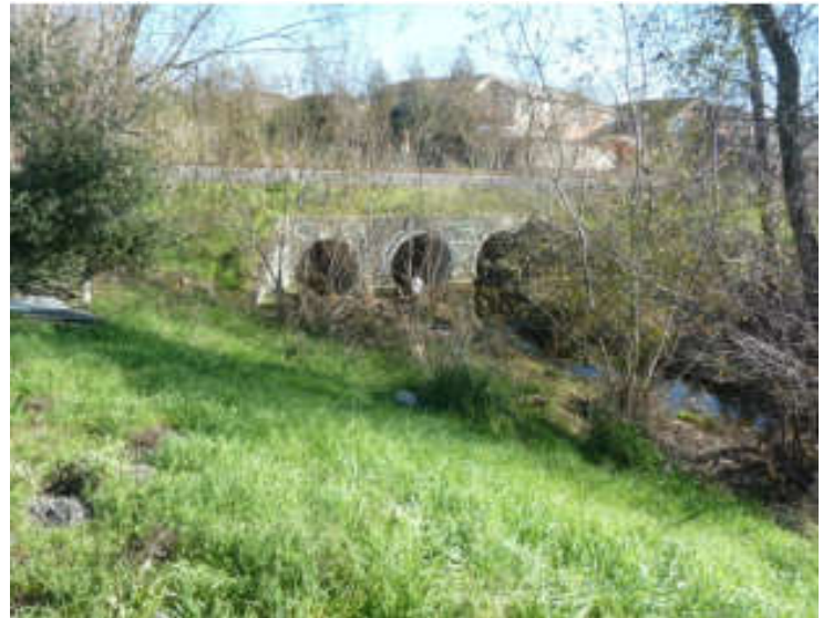
Photo #8: Southeastern adjoining property (creek & culvert)
