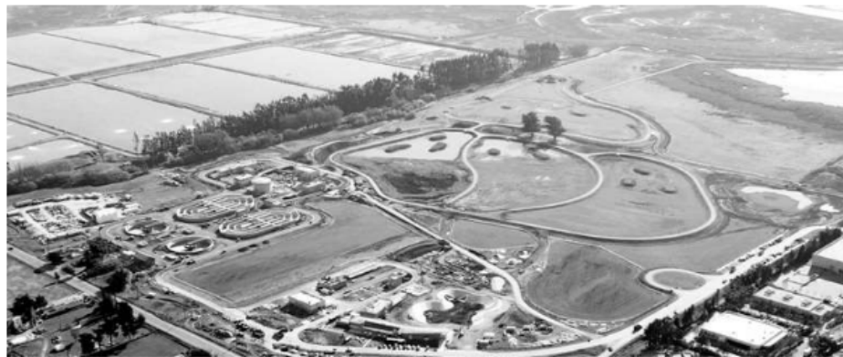
The Ellis Creek Water Recycling Facility, nearing completion, will provide tertiary recycled water to offset potable demand.
