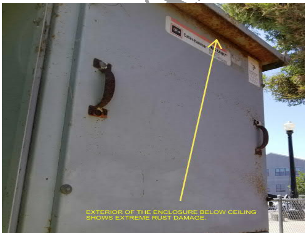
Photo E- 3 Exterior Service Entrance Switchboard Enclosure Ceiling
