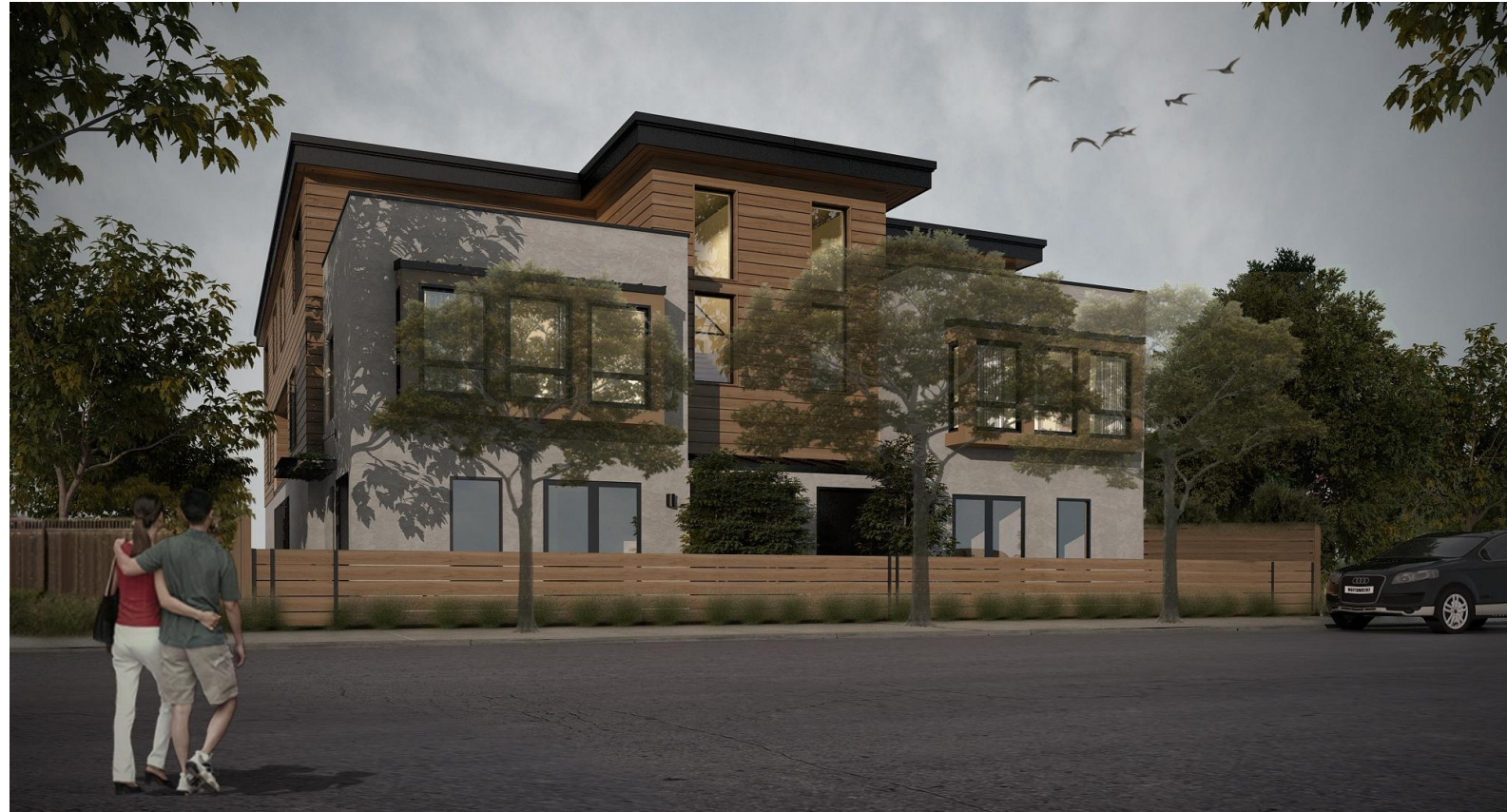
VIEW FROM LAKEVILLE STREET
