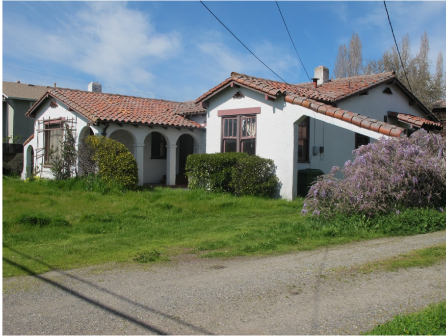
Figure 1 Building A - Looking North
