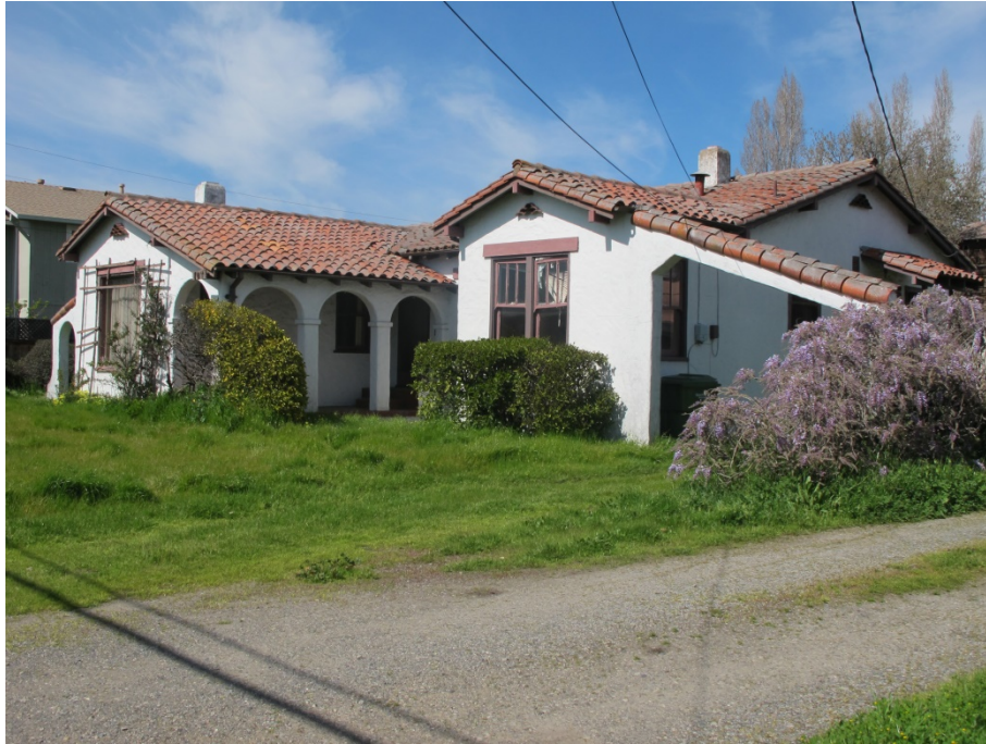
Figure 1 Building A - Looking North
