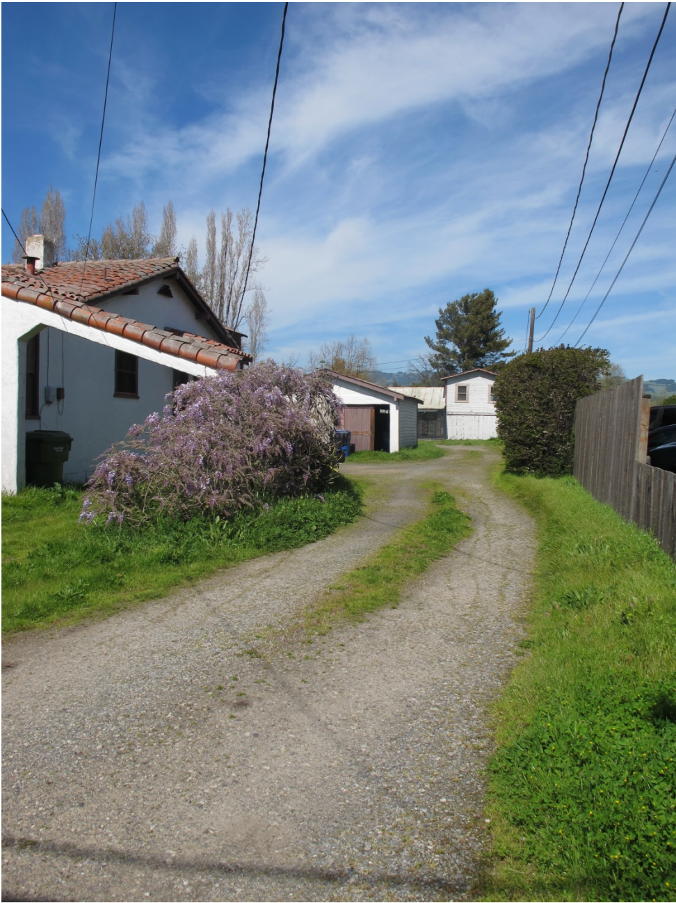
Figure 5 Structure 1 (garage)- Looking North
