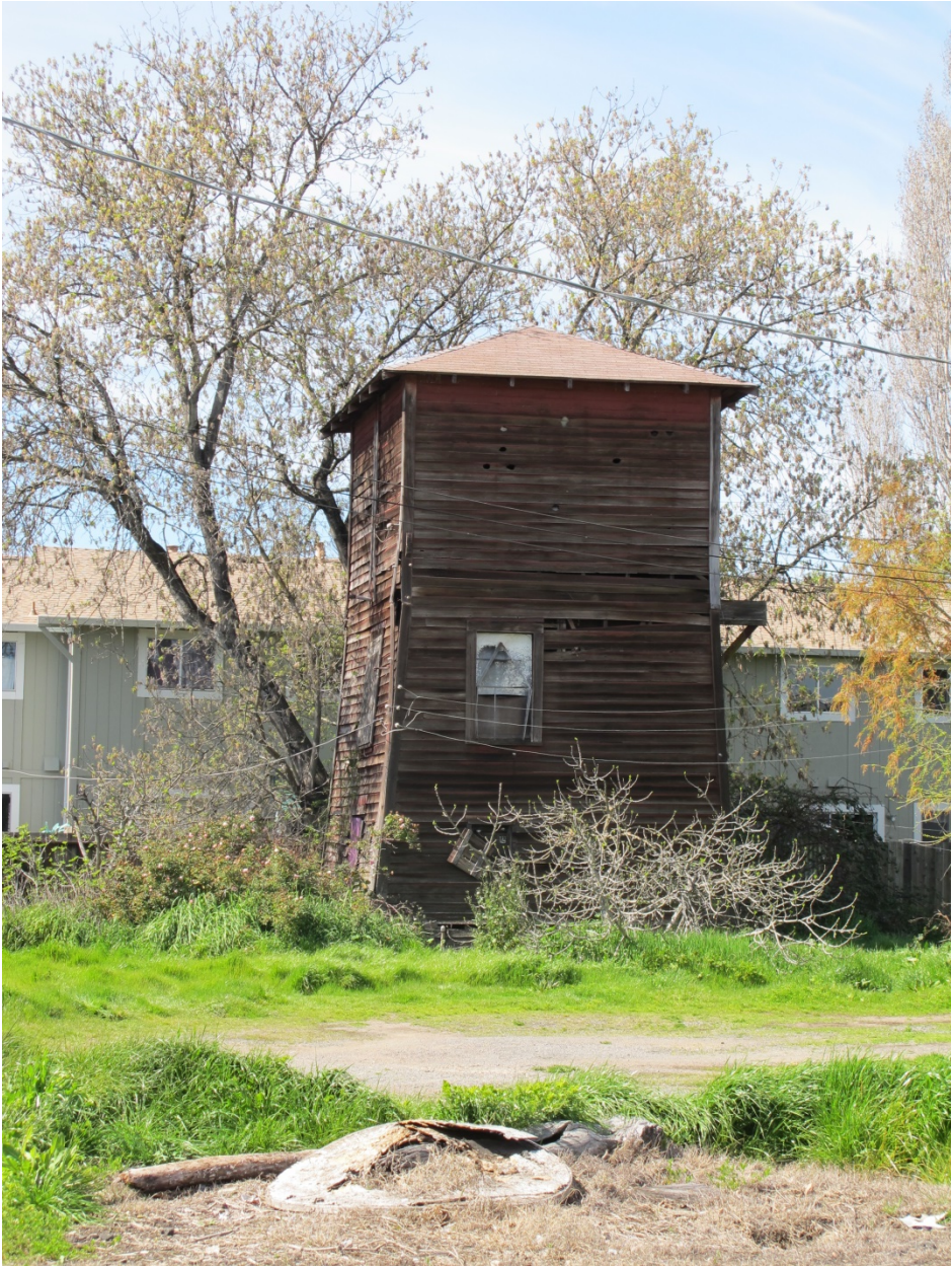
Figure 6 Structure 2 (tank house)- Looking Northwest
