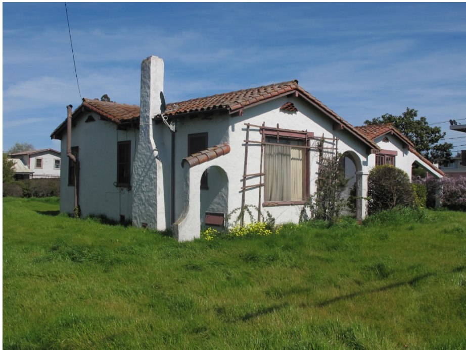
Figure 2 Building A - Looking Northeast
