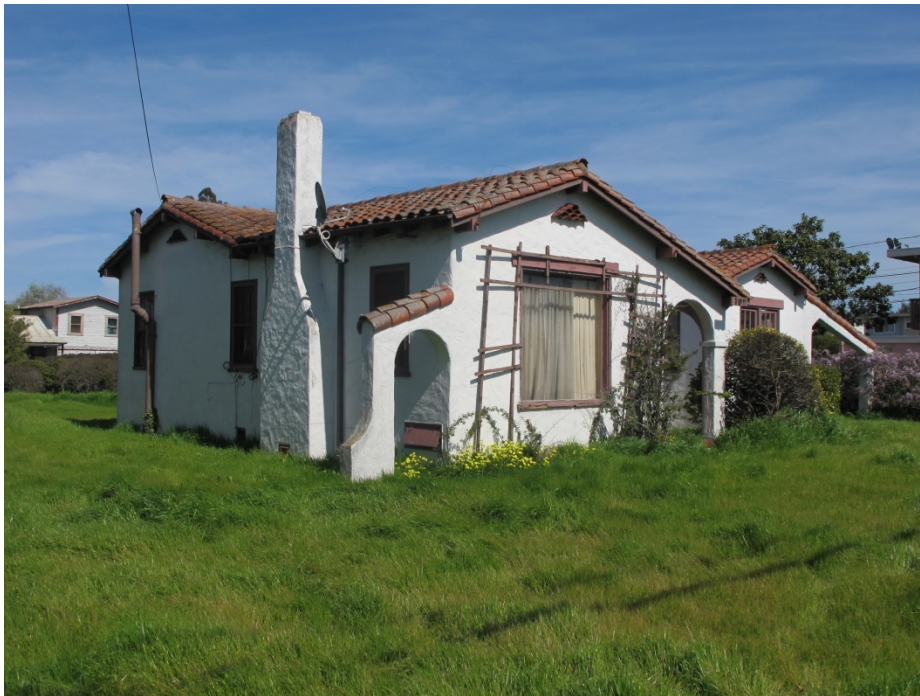
Figure 2 Building A - Looking Northeast
