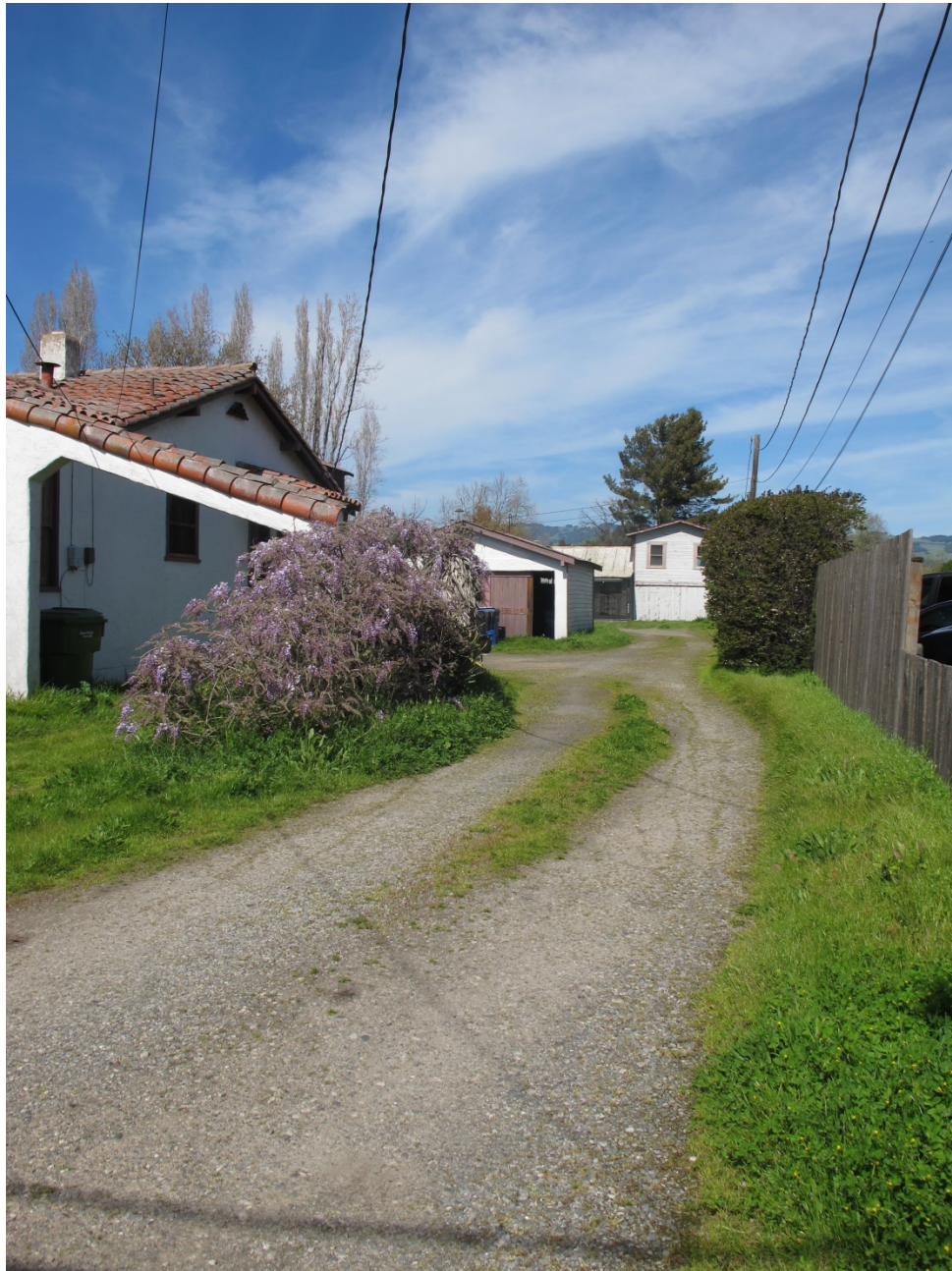
Figure 5 Structure 1 (garage)- Looking North
