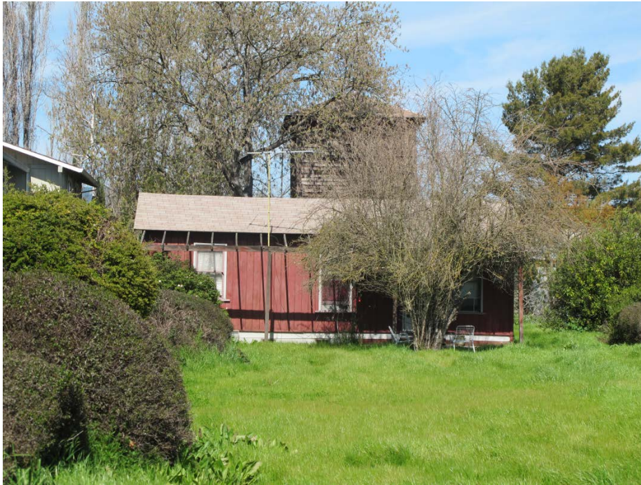
Figure 3 Building B- Looking Northeast
