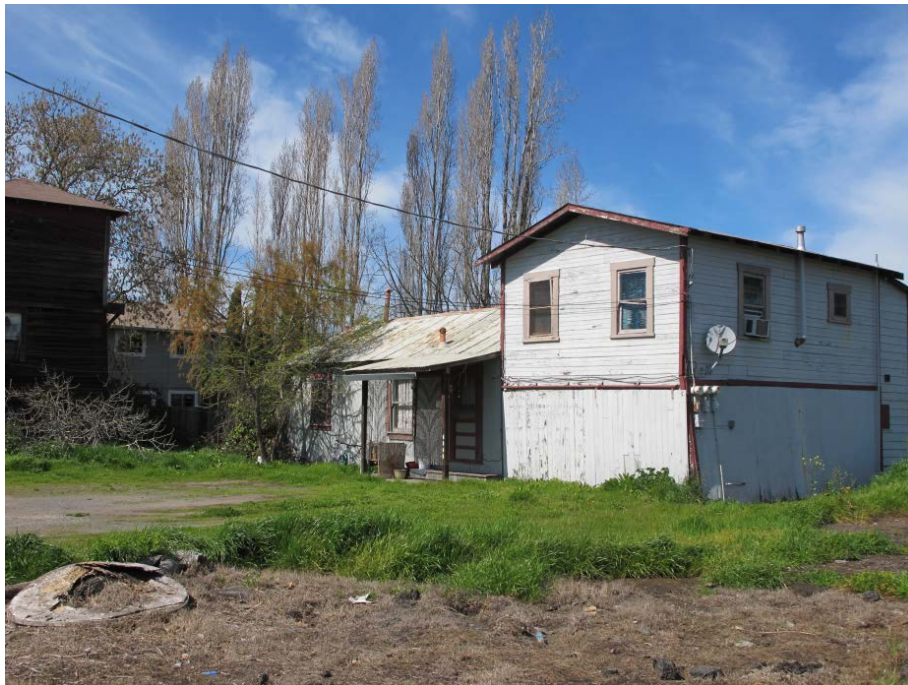
Figure 4 Building C- Looking North
