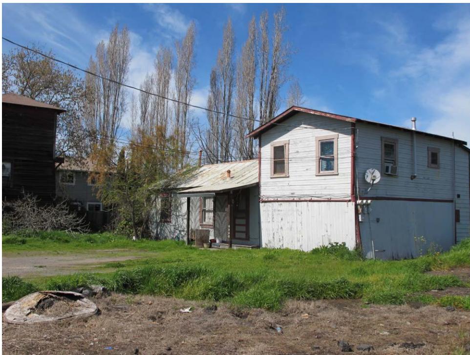
Figure 4 Building C- Looking North
