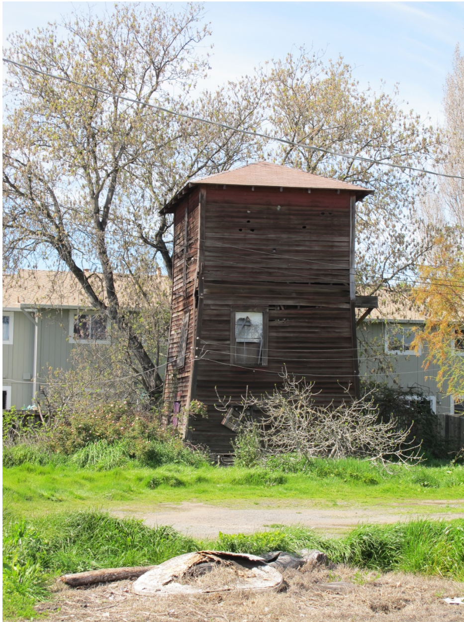
Figure 6 Structure 2 (tank house)- Looking Northwest
