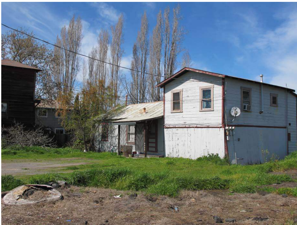
Figure 4 Building C- Looking North
