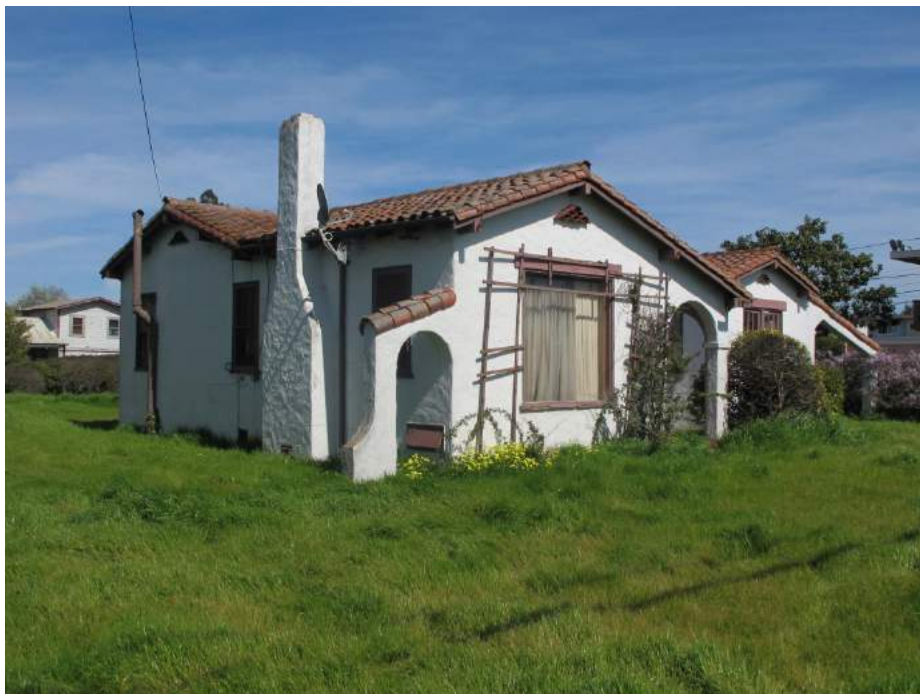
Figure 2 Building A - Looking Northeast
