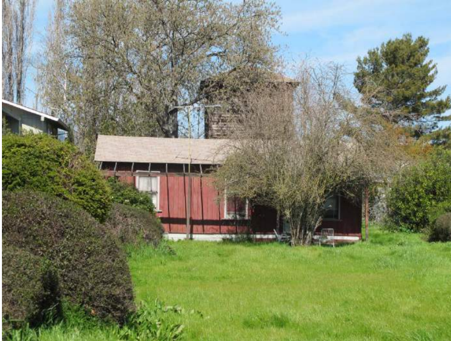
Figure 3 Building B- Looking Northeast
