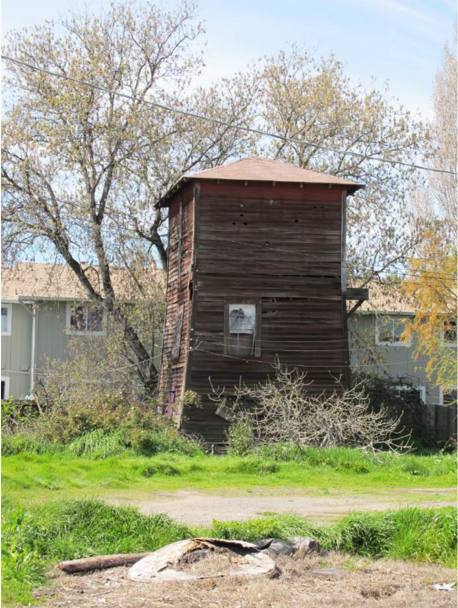
Figure 6 Structure 2 (tank house)- Looking Northwest
