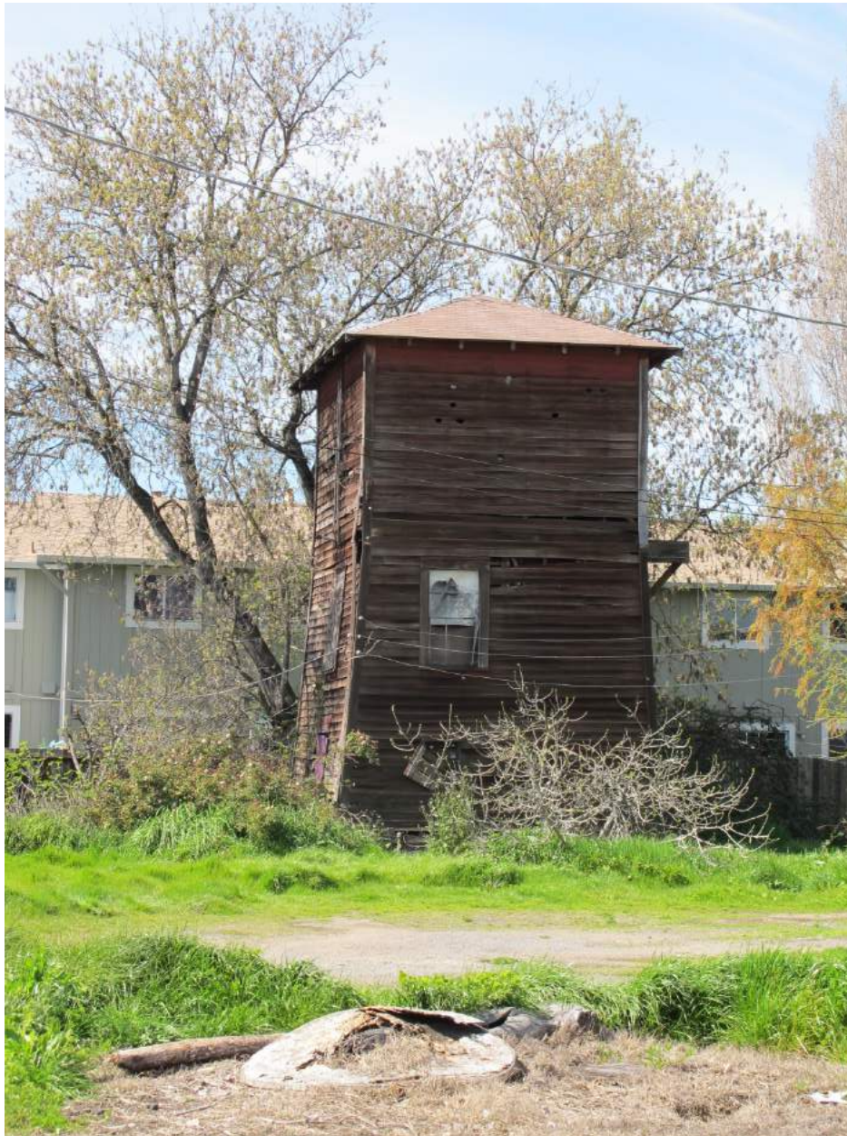
Figure 6 Structure 2 (tank house)- Looking Northwest
