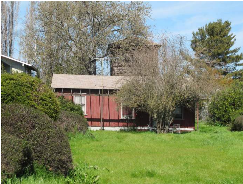
Figure 3 Building B- Looking Northeast
