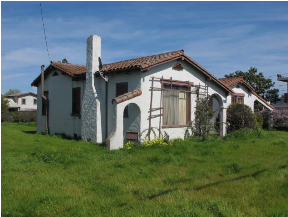
Figure 2 Building A - Looking Northeast
