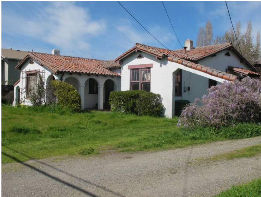
Figure 1 Building A - Looking North
