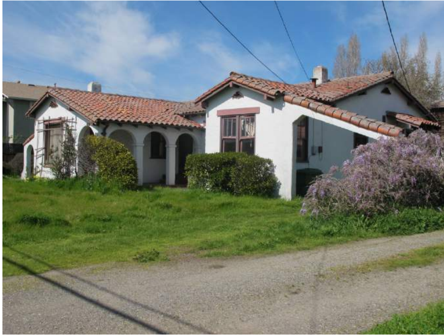
Figure 1 Building A - Looking North
