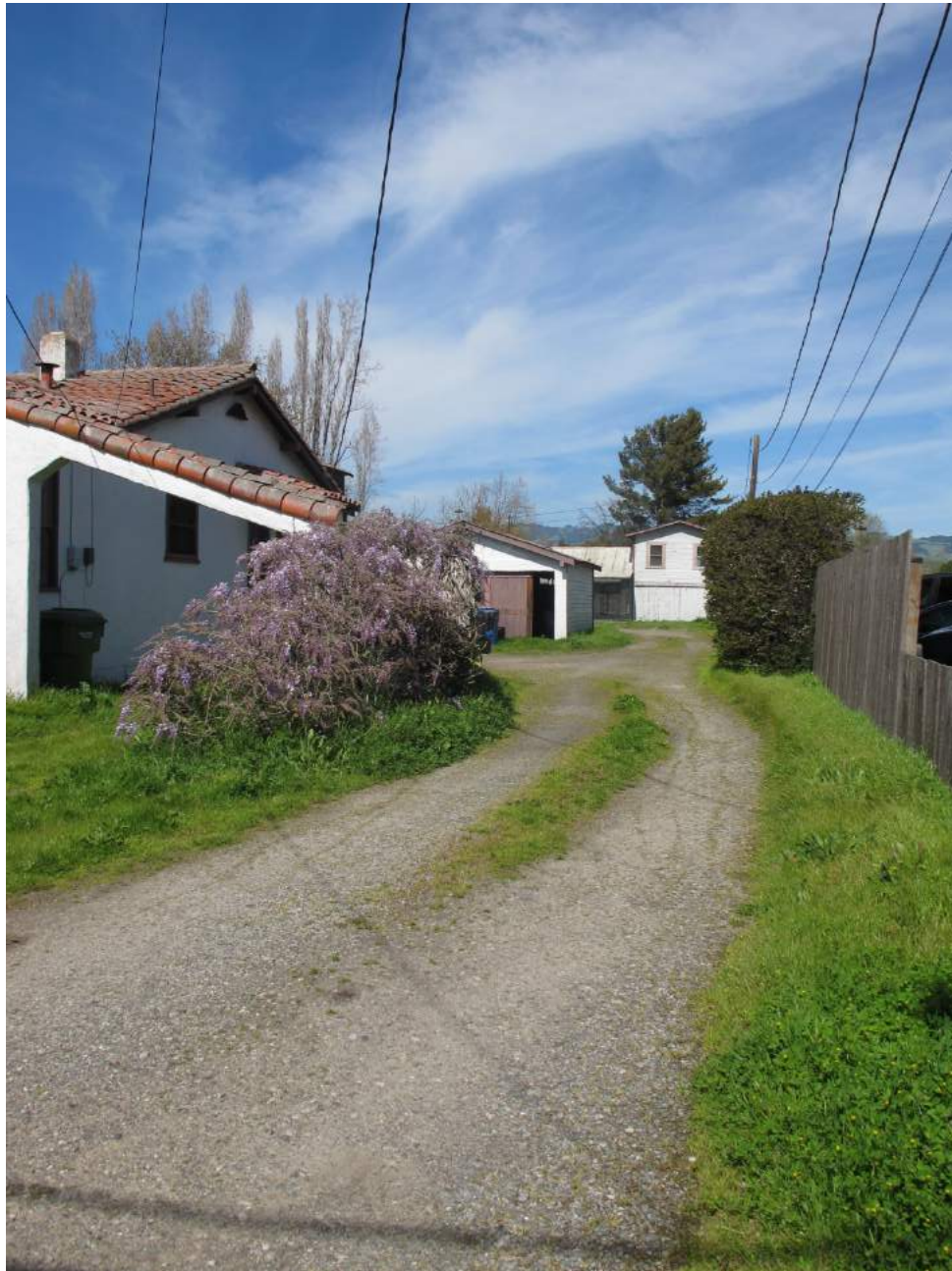
Figure 5 Structure 1 (garage)- Looking North
