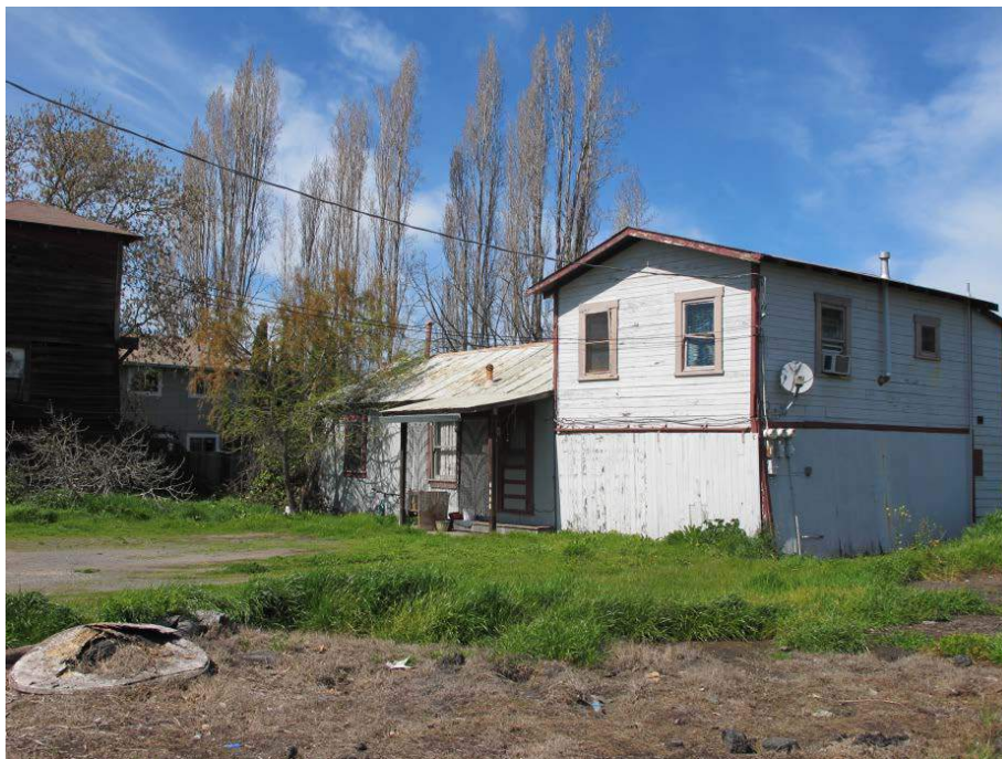
Figure 4 Building C- Looking North
