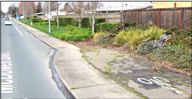
16 – Beyond Rainier – widening for bike lane
