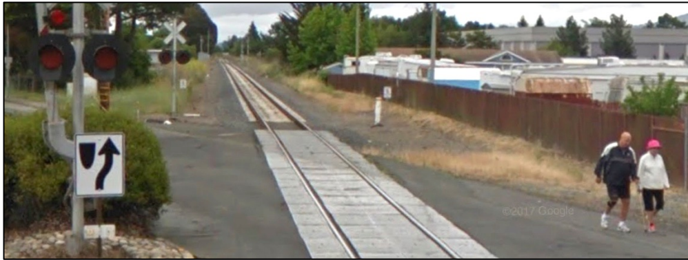
a) Rubber grade crossing panels; 2 northbound pedestrians on south side
