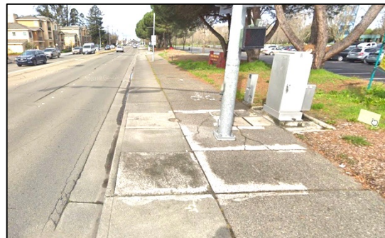
4 – Community Center Way
