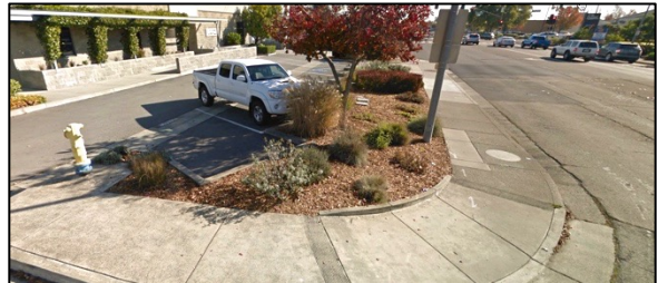
2 - Public Works north driveway, facing south
