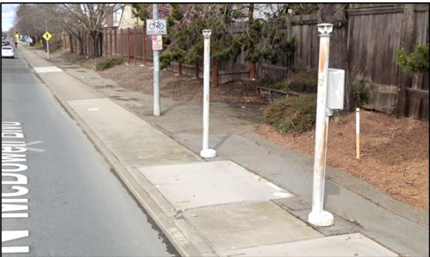
18 – Vent pipes north of Cottages
