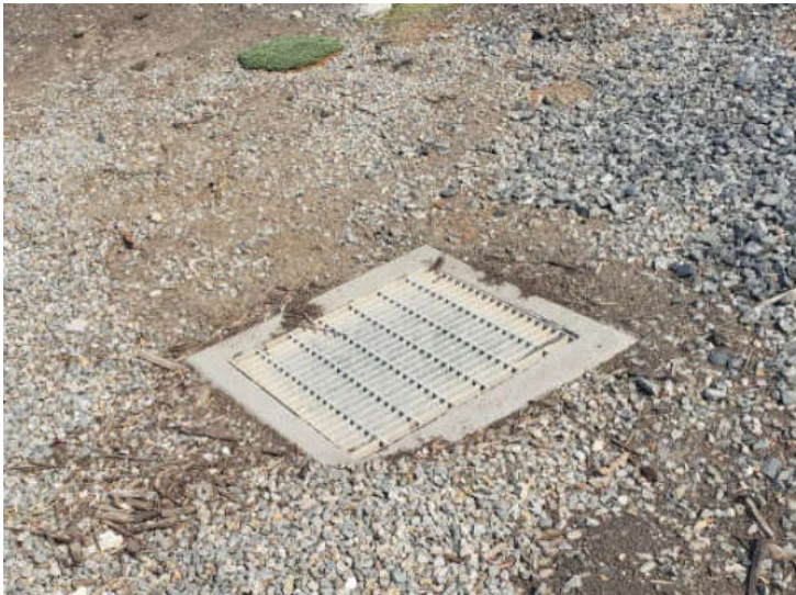
Photo #22: Grated stormwater drain on southern border
