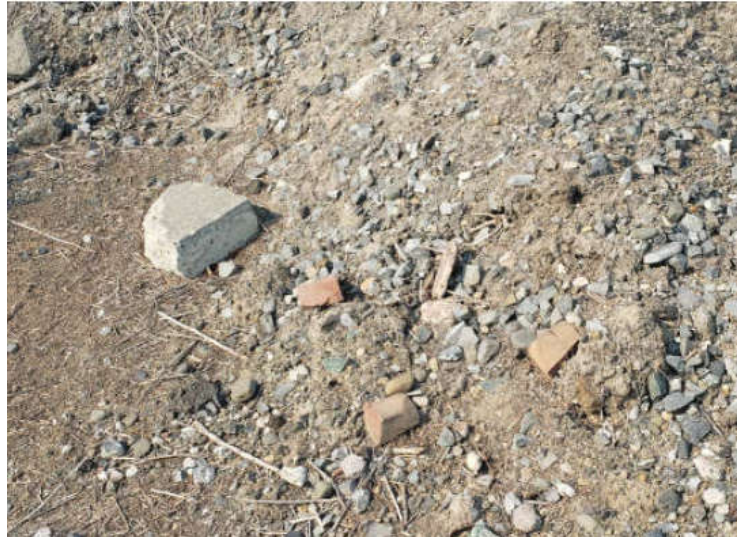
Photo #20: Typical concrete and brick debris in soil pile
