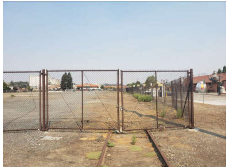
Photo #11: Railroad tracks terminus and northeastern gate entrance
